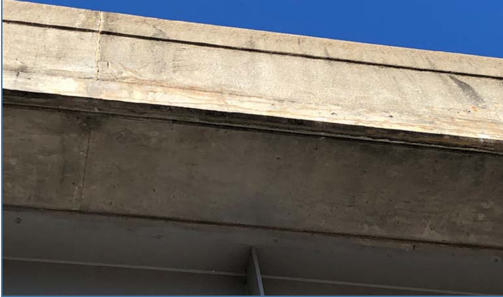
Photo 29: 12/23/2019 A2942: Rte. 21 NB over Old Rte. 21 Left barrier curb, horizontal cracking
