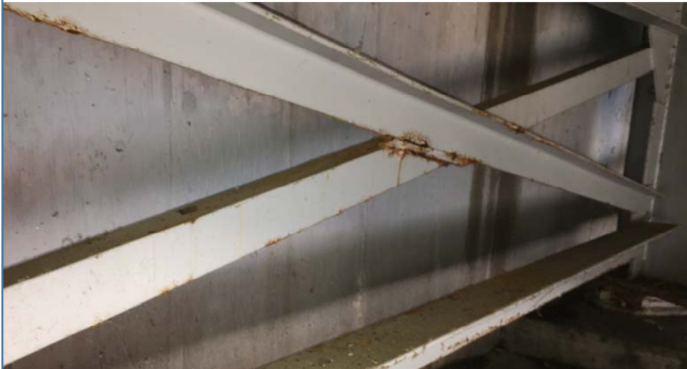
Photo 15: 11/19/19 A3100: Old Rte. 21 over Rte. 21 Typical rust on cross-frame at EB1&5 between G2&3-EB1, G4&5-EB1, G2&3-EB5
