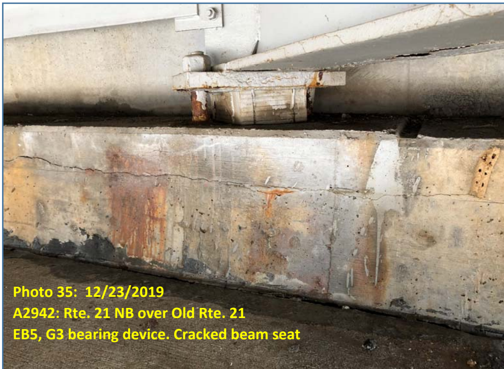
Photo 36: 12/23/2019 A2942: Rte. 21 NB over Old Rte. 21 EB5, G3 bearing device. Cracked beam seat
