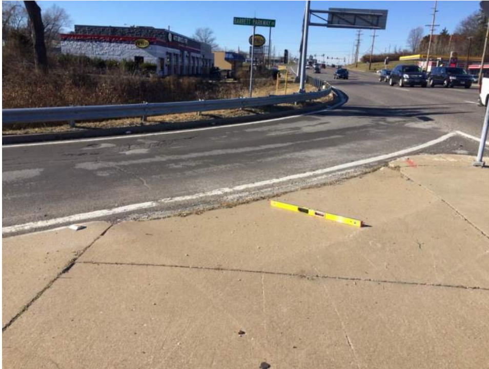
Sidewalk ramp with no warnings and no receiving ramp on opposite side.
