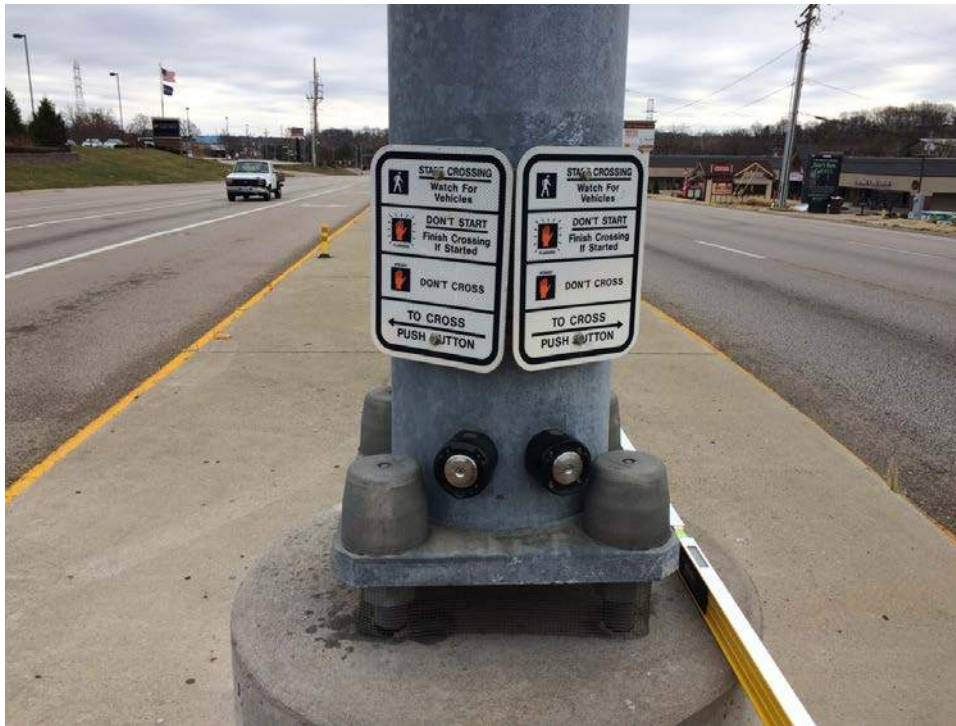
Pedestrian buttons not 10 feet apart.
