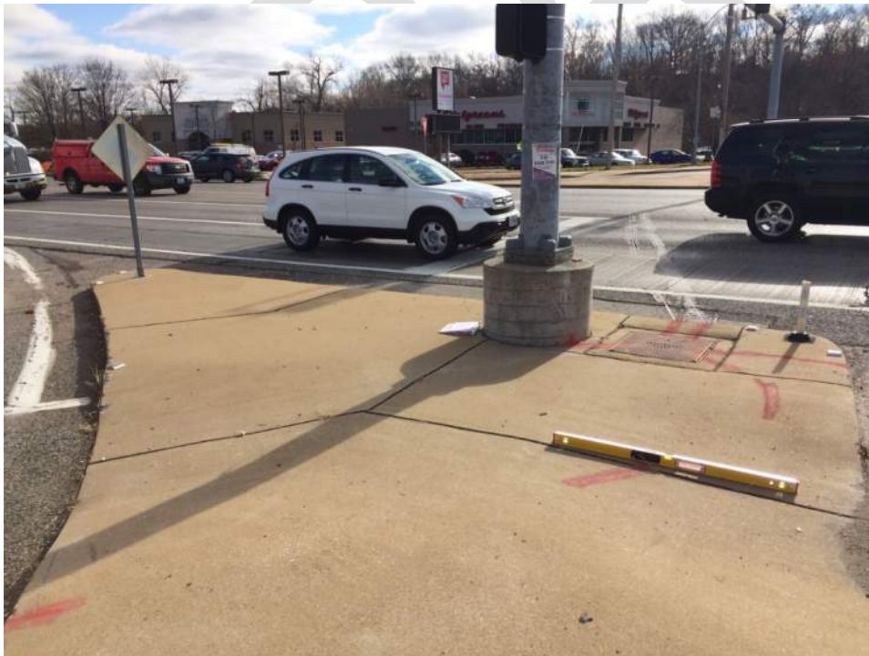
No detectable warnings or pedestrian buttons. Steep ramp grades.
