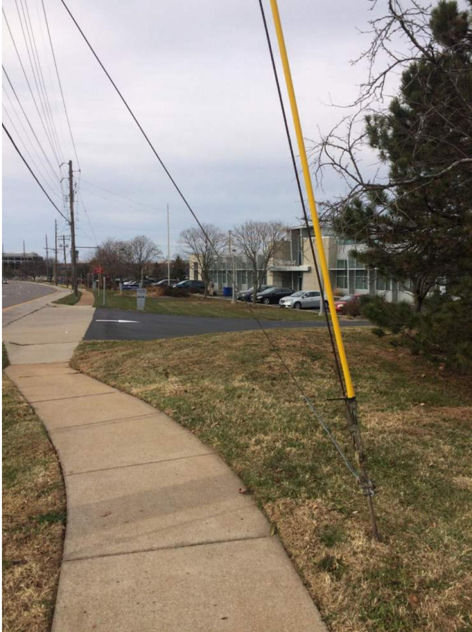
Vertical encroachment due to guy wire.
