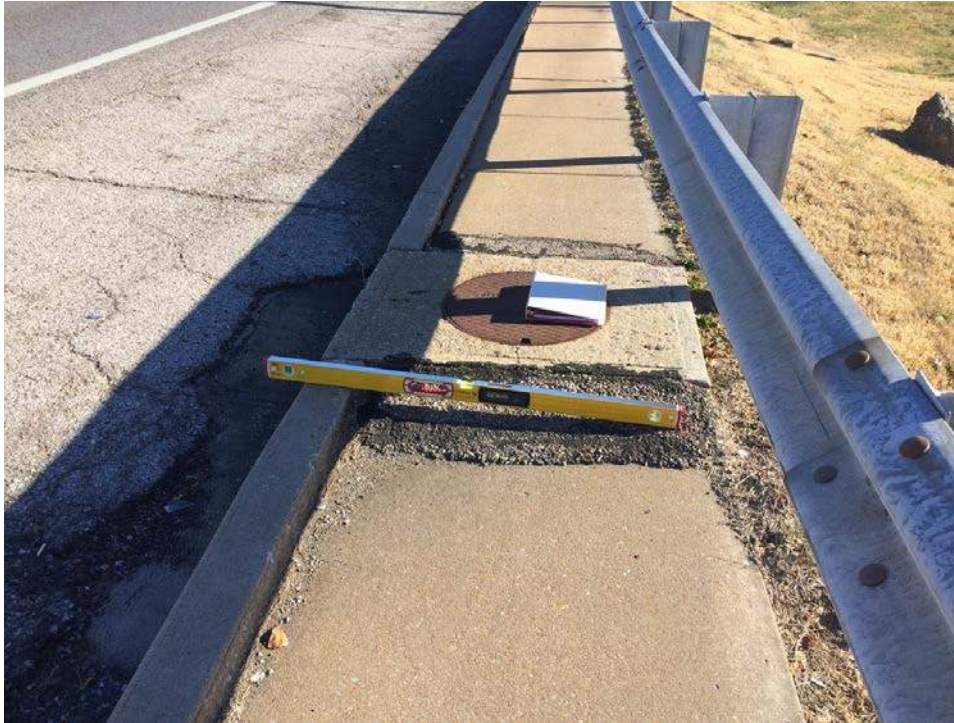
Sidewalk width less than 4 feet and trip hazards.
