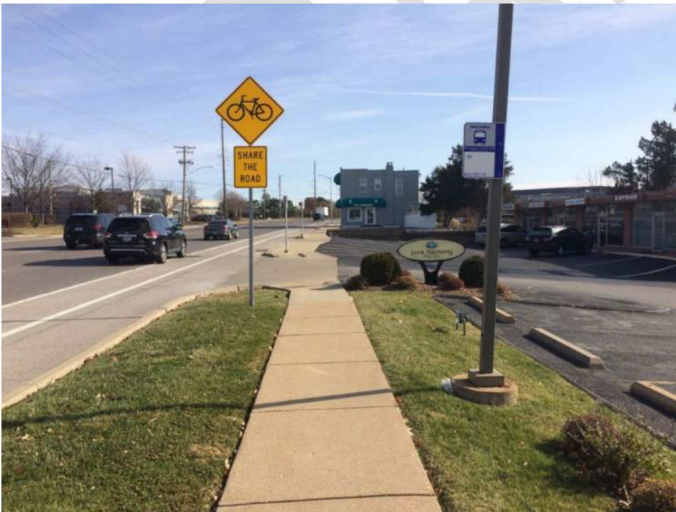
Bus Stop Sign Only, sidewalk present but not connected to back of curb.
