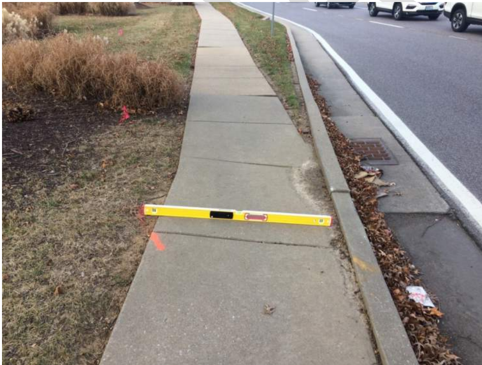
Excessive cross slope and trip hazards.
