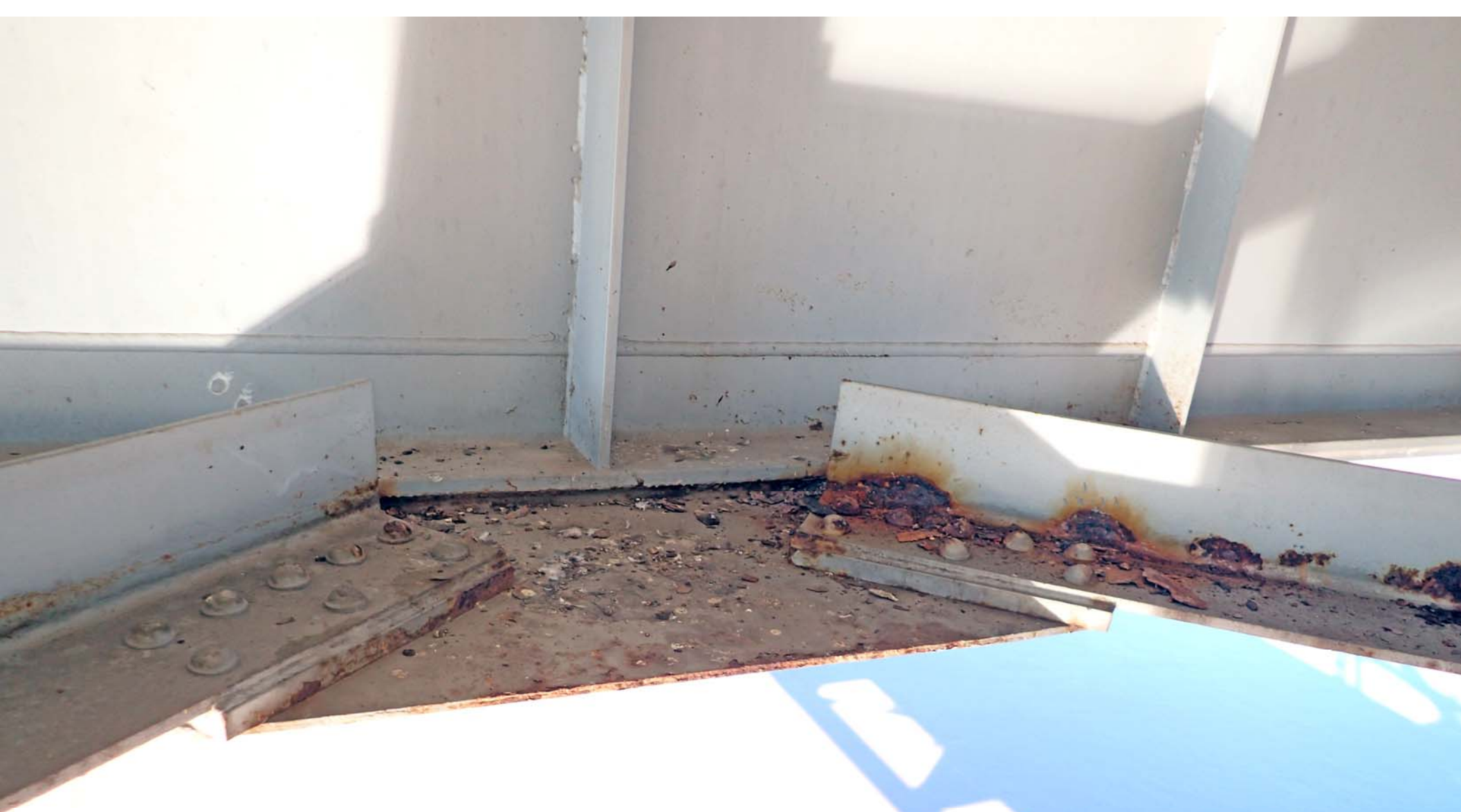
L0962 I-70 Cooper Floorbeam L7'L7' Middle X-brace Gusset Plate and Member Section Loss 8-29-17
