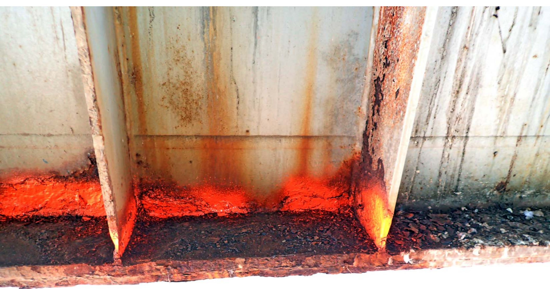
L0962 I-70 Cooper Floorbeam L12'L12' Stringer 5 Saddle Bearing Support Moderate Section Loss 8-29-17
