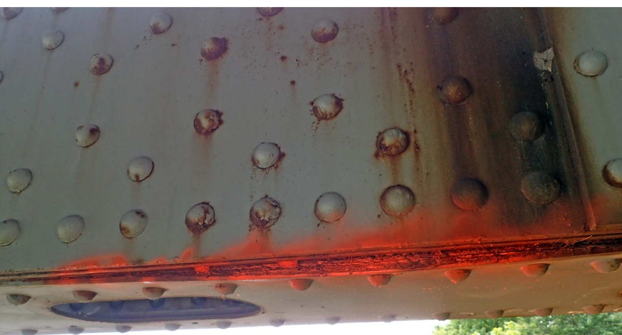
L0962 I-70 Cooper East Truss Lower Chord L4L5 Bottom Plate Packrust Distortion (typ) 8-30-17
