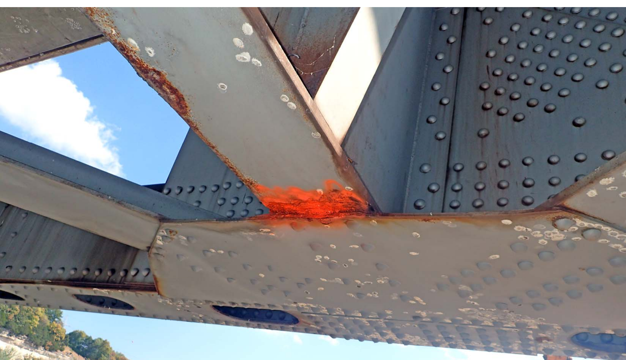
L0962 I-70 Cooper Floorbeam L16'L16' East End Bottom Flange Heavy Section Loss 10-2-17
