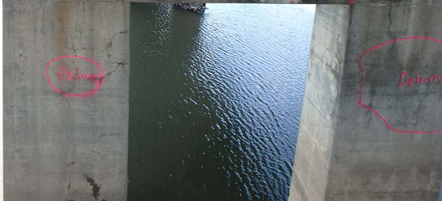
L0962 Cooper 70 8/28/17 Bent 7 east side capface all delaminated with hvy spalling with rebar exposed
