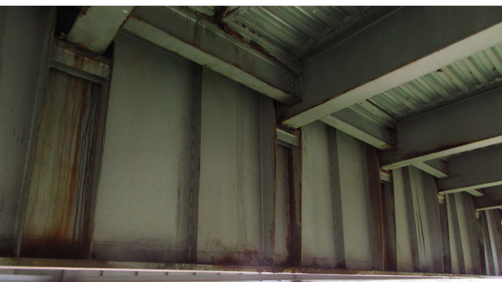
L0962 Cooper 70 E 8/24/15 Span 13 L4 floorbeam west side with moderate pack rust in web and bottom flange under stringer 5 saddle bearing
