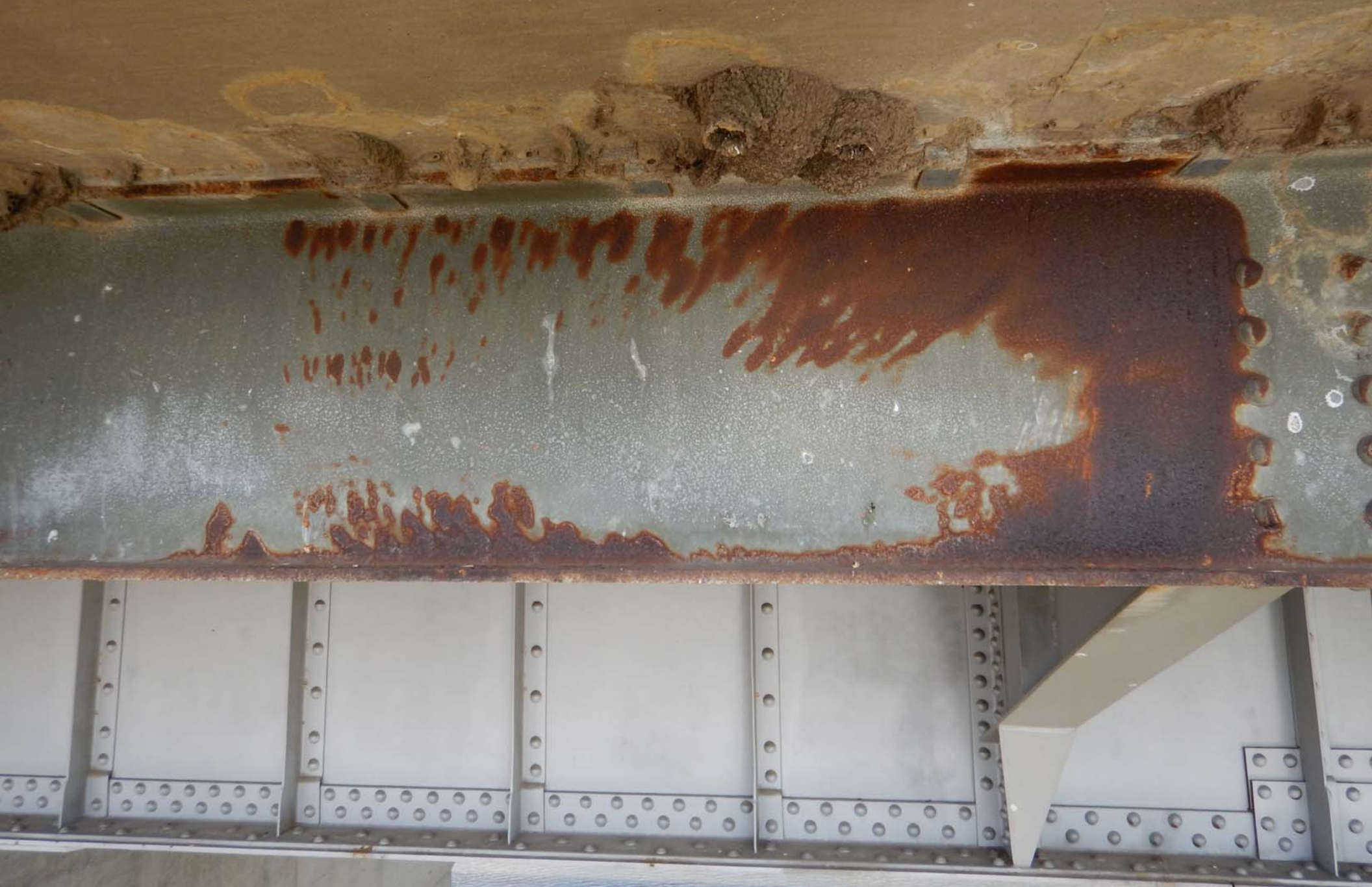
L0962 Cooper 70 9/10/15 Span 8 outside stringer south side with minor rusting
