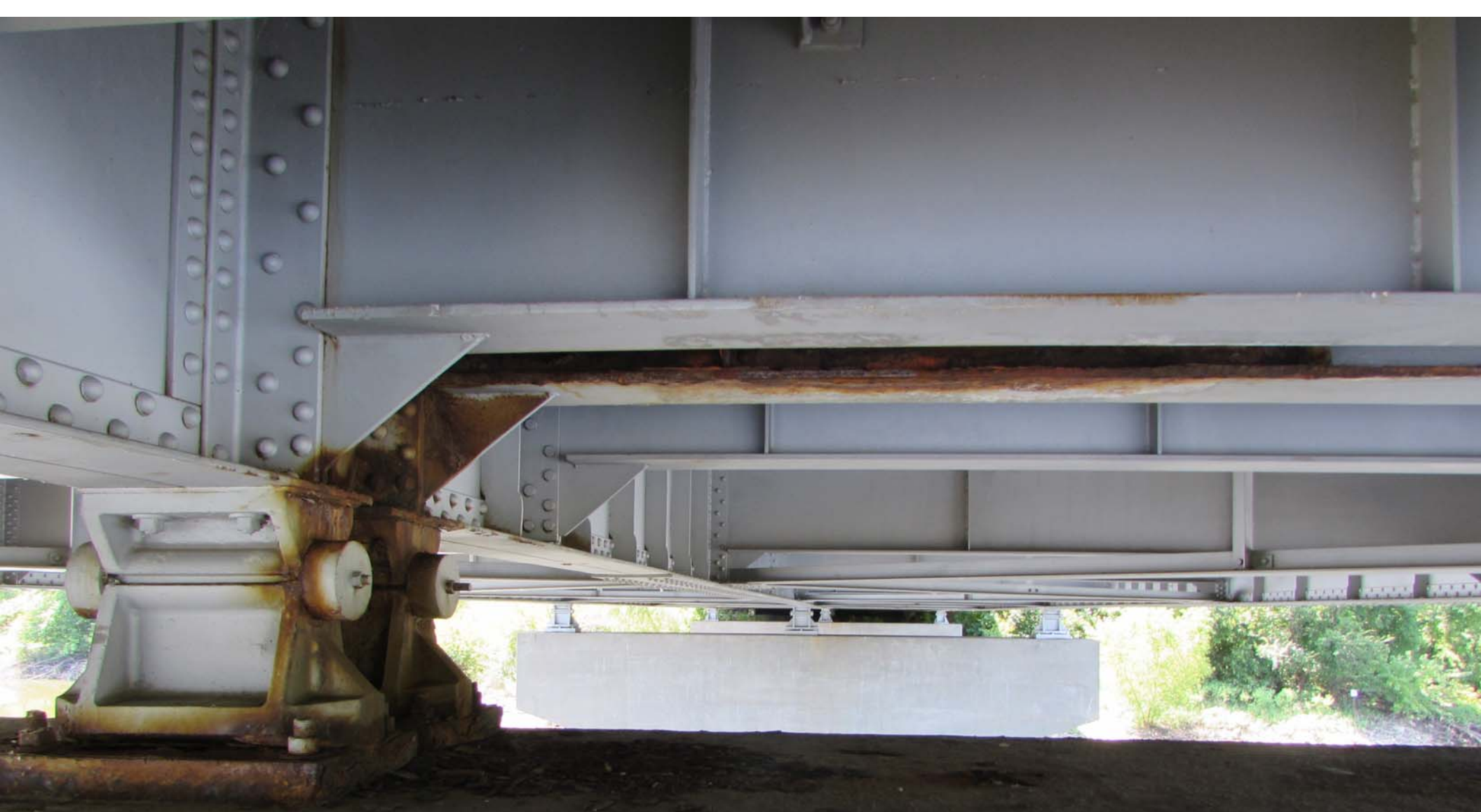
L0962 Cooper 70 E 8/24/15 Bent 4 rockers and floorbeam with hvy pack rust and sec loss with 50 percent remaining
