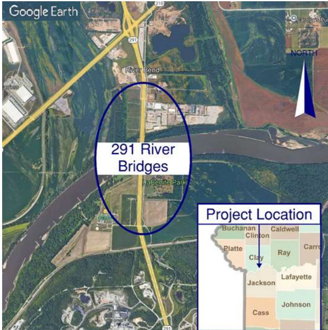
Missouri Route 291 Bridge over the Missouri River in Jackson County
