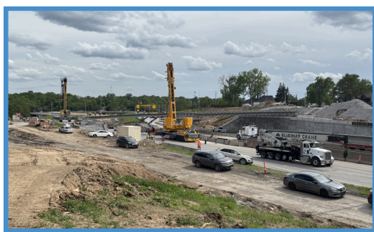
Girder installation at 27 th St. bridge
