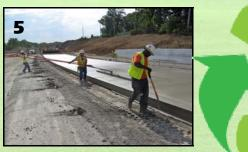
The crushed concrete is then used as an aggregate base that lies beneath the concrete pavement that we drive on.
