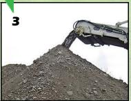
The rubble is loaded into large portable crushers that can crunch up to 600 tons of concrete per hour.
