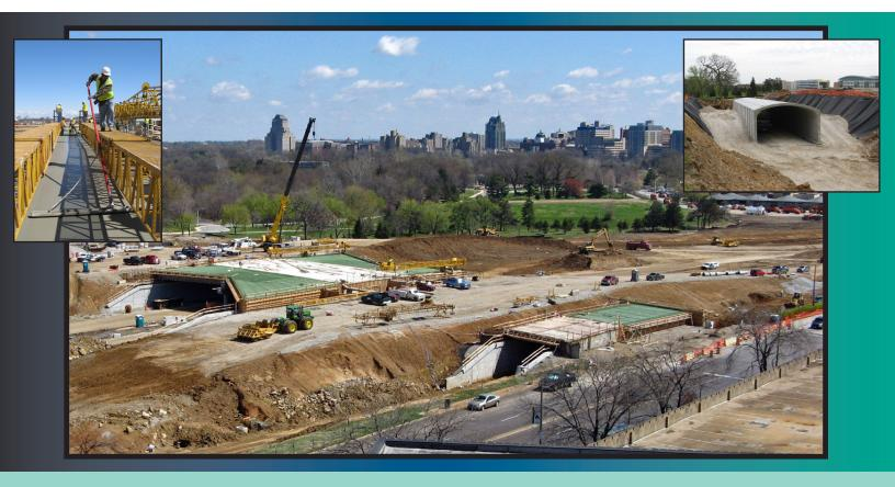
ABOVE: The Hampton Avenue bridge over I-64 takes shape by Forest Park. Bridge deck paving is nearly complete and the structure is on schedule to open one lane in each direction by May 22. A new roundabout at the Hampton/Wells Drive intersection will open at the same time. A new underpass for the bike and pedestrian trail now crosses under Hampton in Forest Park.
