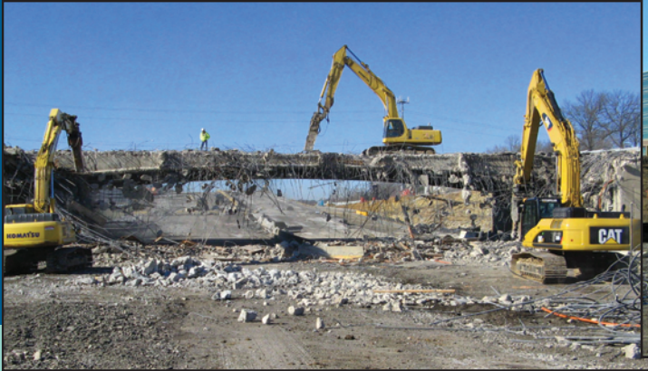
ABOVE: Demolition begins on the eight-month reconstruction of the Hanley Road bridge over I-64. For an illustration of the Hanley detour route, see page four. BELOW LEFT: Concrete from demolished bridges and pavement is crushed and turned into fill material for new roadbed near Laclede Station Road. BELOW MIDDLE & RIGHT: Demolition of the I-64 bridge over Claytonia Terrace will close that street for as long as 90 days. A total of nine structures will be rebuilt on the second half of the project.
