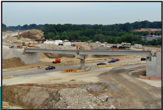
Girders are in place over Brentwood Boulevard for what will become the south-to-west flyover ramp from I-170 to I-64.
