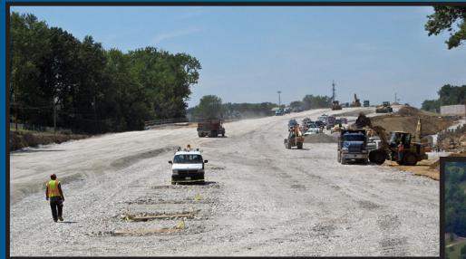
A massive grading and fill operation east of the Lindbergh Boulevard interchange filled in a large dip in the road. Most of the roadbase you see in this photo is recycled concrete from the old highway and bridges. RIGHT: An aerial view of the Lindbergh interchange, looking north.
