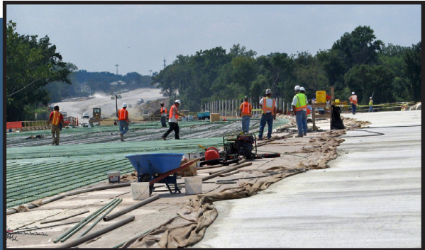
TOP: On the Clayton Warson bridge, crews remove wet burlap used to regulate the speed of the concrete curing process. BELOW: An aerial view of the Clayton Warson bridge looking to the southwest.
