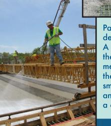
Paving the bridge deck at Lindbergh. A pump truck pours the concrete over a mesh of steel rebar, the surface is then smoothed, grooved, and sprayed with a curing compound.
