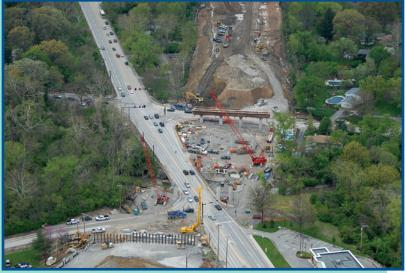
At the I-64 bridge over Clayton and Warson Roads lots of construction activity and live traffic share a very small area. By the end of May the first of 90 concrete girders will be set to form the bridge deck.
