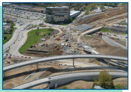
With the completed half of the I-170/I-64 interchange at the bottom of the photo, the two remaining flyover ramps and the I-64 bridge over Brentwood Boulevard can be seen taking shape next to the Magna Building.
