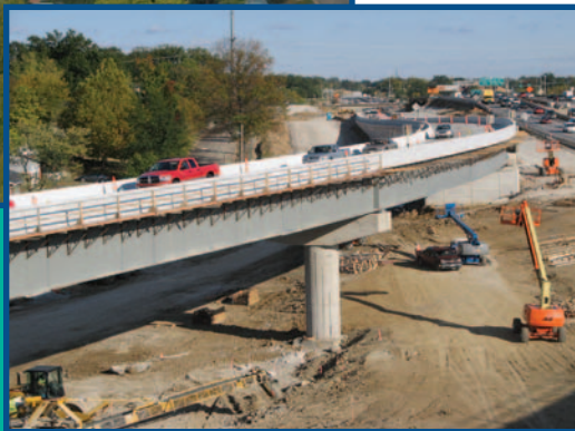
ABOVE: Construction continues on the flyover ramps for the freeway-to-freeway interchange connecting I-170 with I-64. RIGHT: Traffic is already using the westbound to northbound ramp.
