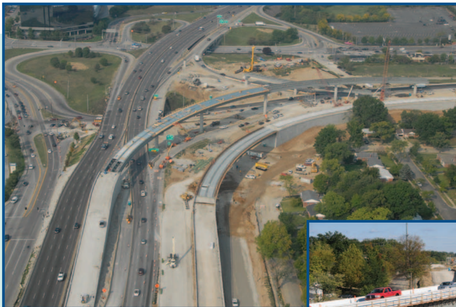
ABOVE: Construction continues on the flyover ramps for the freeway-to-freeway interchange connecting I-170 with I-64. RIGHT: Traffic is already using the westbound to northbound ramp.
