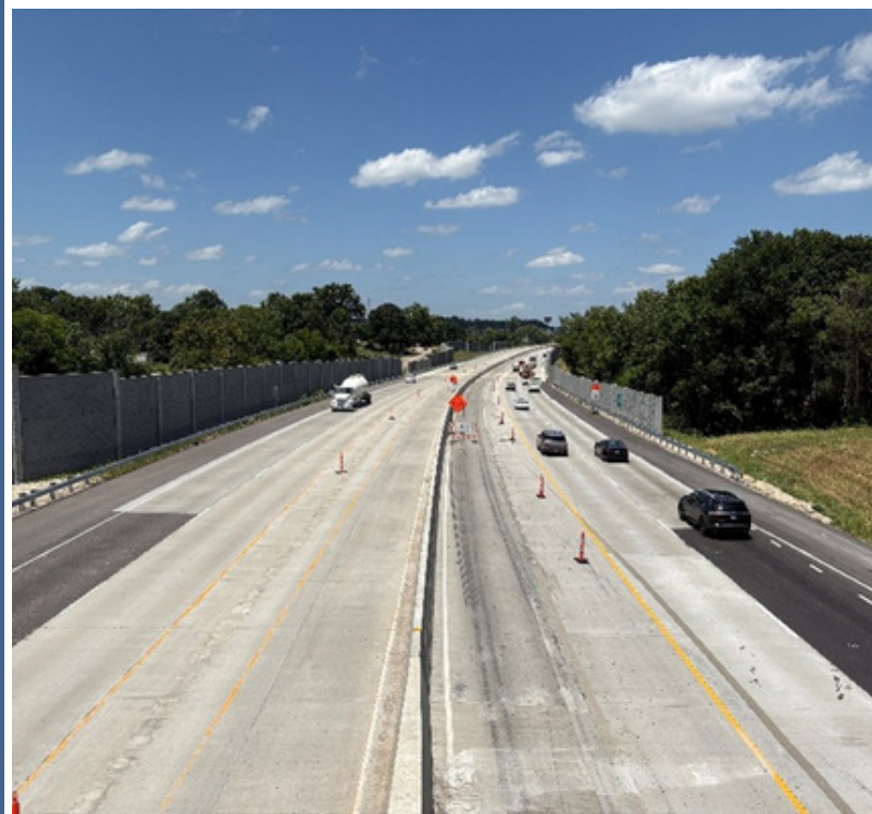
Temporary barrier recently removed from I-55 north of Main St.
