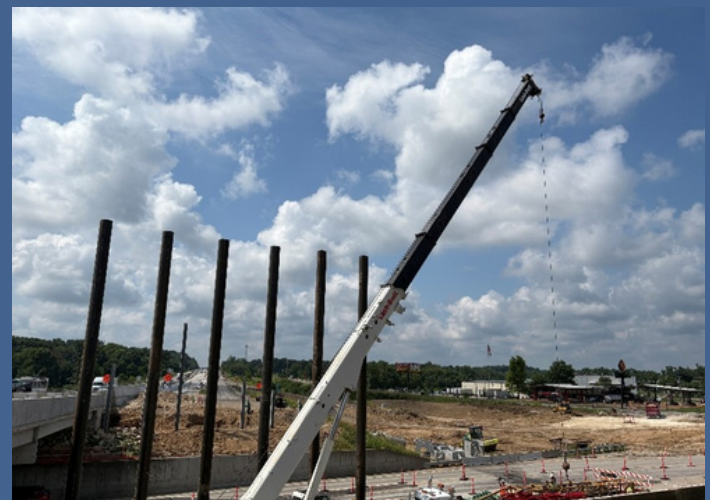
Pile being set for new southbound I-55 over Route Z
