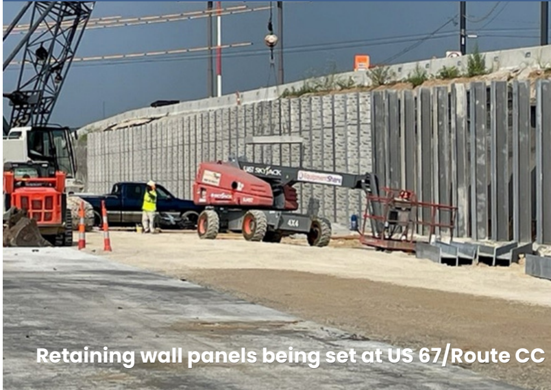
Retaining wall panels ready to set at US 67/Route CC
