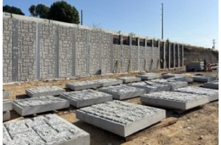
Retaining wall panels ready to set at US 67/Route CC
