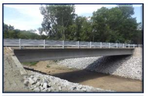
Mercer County Bridge #01300062, BRO-B065 (37)This is a 92' long single span, concrete girder bridge. Constructioncost was \$310,618. Construction was completed Summer.Reference:Shane Grooms, Associate CommissionerPhone:(660) 748-3425
