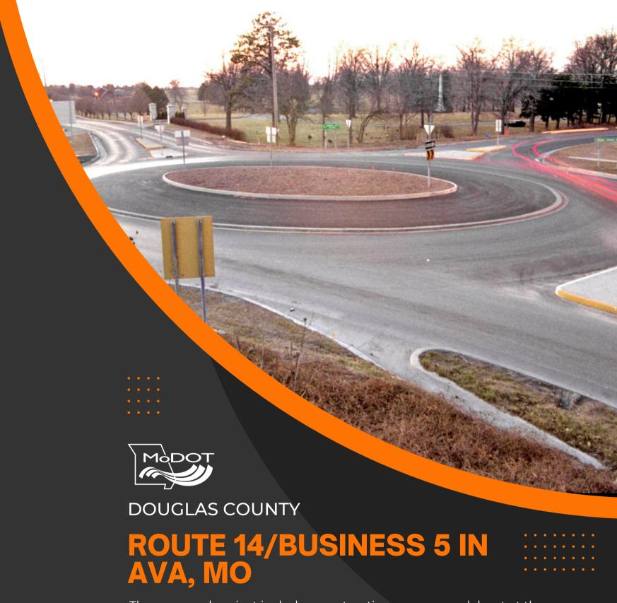
The proposed project includes constructing a new roundabout at the intersection of Route 14, Business 5, N. Jefferson St., and Bacorn Ave. This project will also include drainage and pedestrian improvements in the vicinity of the proposed roundabout. The proposed roundabout will have designated pedestrian crossings on N. Jefferson St. and Bacorn Ave.
