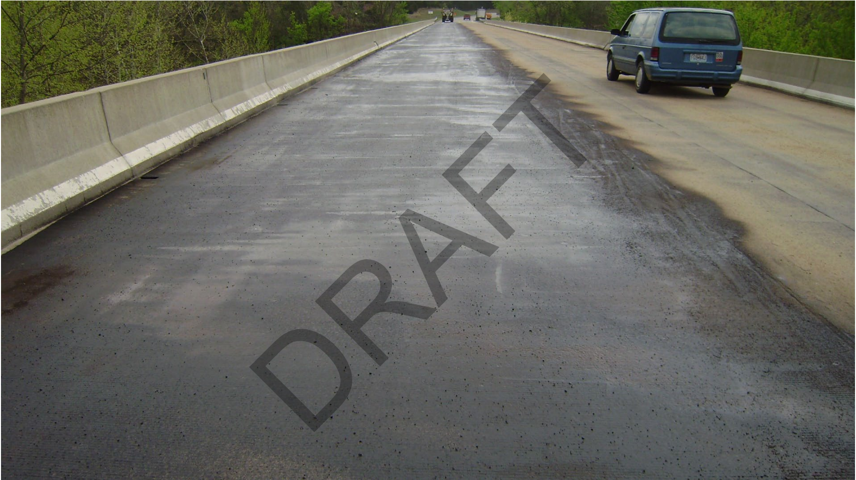
Typical bridge deck seal
