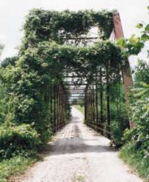
The Bonanza Bridge in Caldwell County before adaptive reuse.
