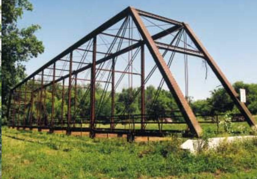
The Bonanza Bridge after it was saved from the scrap heap.
