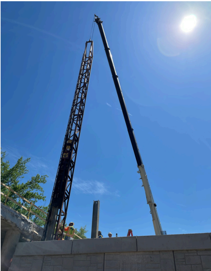
Pile being driven for south abutment of 3rd Street bridge
