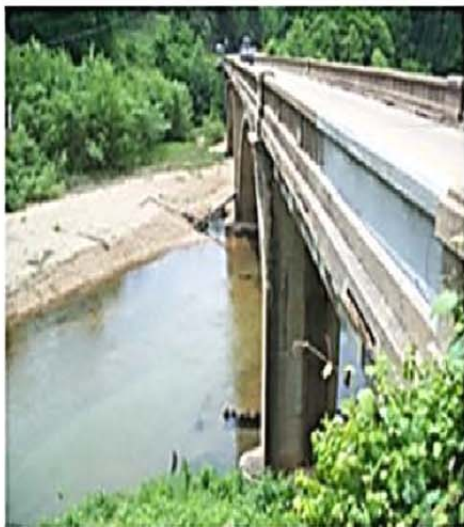
East side of bridge, South approach
