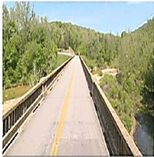
On the bridge, looking north
