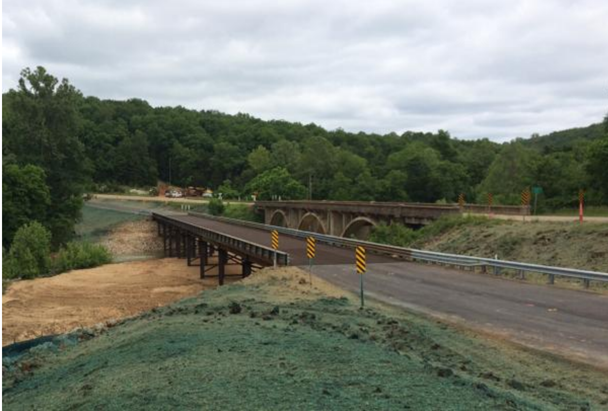
Figure 5: Temporary Bridge Photo
