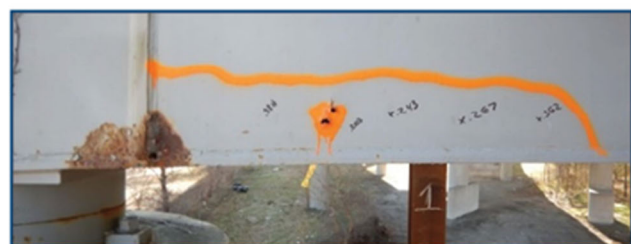
Area of Section Loss
