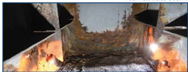
Section Loss from Inside
