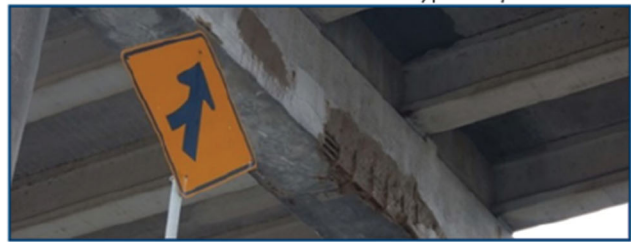
Typical Cast Deterioration
