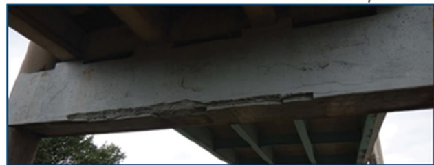
Typical Cap Deterioration
