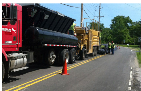
LPA Project West Watson Road – Construction Inspection
