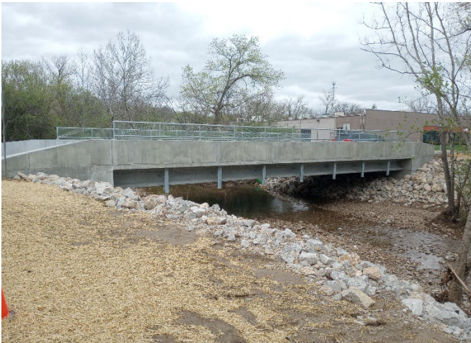
Wyncrest Drive over Glaize Creek – St. Louis County
