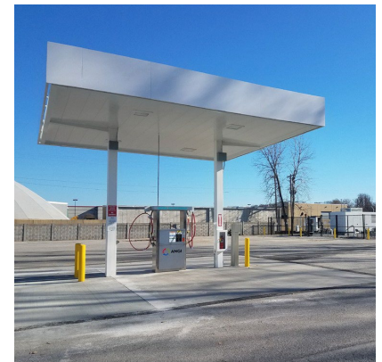
LPA Project CNG Station, Chesterfield, MO Construction Inspection
