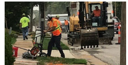
LPA Project N. Geyer Rd. Construction Inspection
