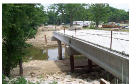
LPA Project Joachim Bridge – Construction Inspection
