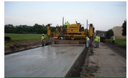
LPA Project Hazelwood Ave. Construction Inspection
