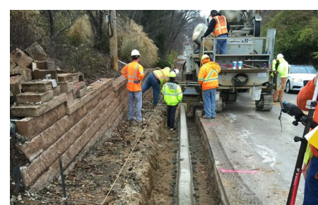
LPA Project Price Road – Construction Inspection
