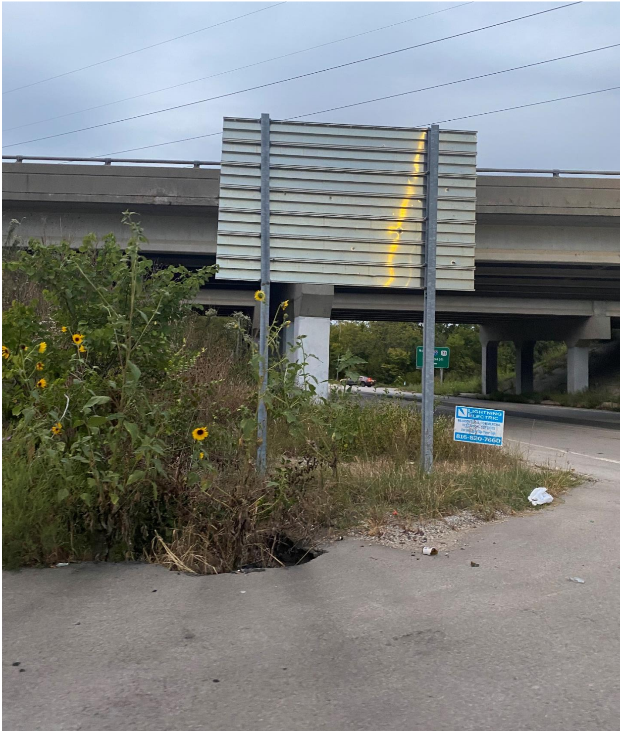
Figure 67: Southbound I-29 Ramp Terminal onto NE Davidson Road
