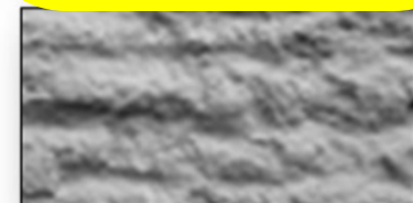
CSP 9 (heavy scarification)
