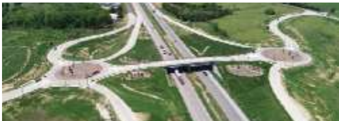
I-70 & Route MM Interchange - Warrenton, MO
