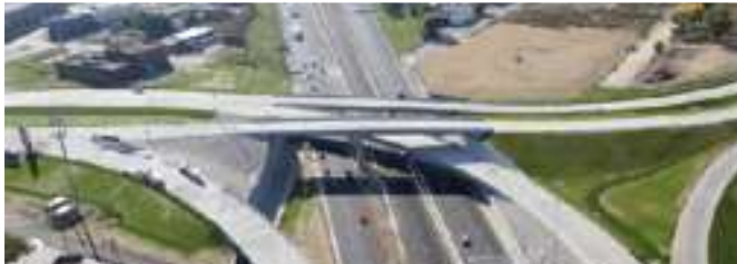
I-70 & Mississippi River Bridge Interchange - MODOT & St. Louis, MO
