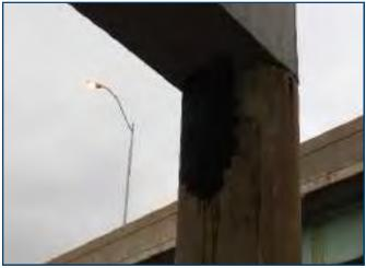
Typical column delamination and spalling with exposed reinforcement.
