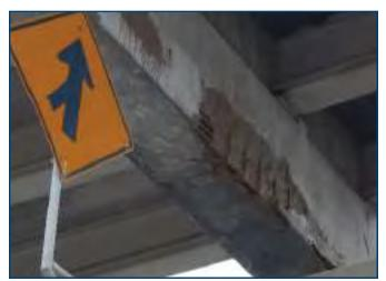
Typical cap under expansion joints with deterioration, delamination, and spalling with reinforcement exposed
