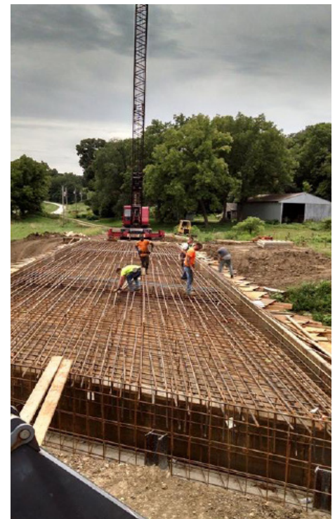
PARK ROAD BRIDGE Cass County, Missouri
