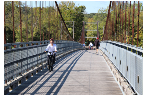
JOE DICE BRIDGE IMPROVEMENT Warsaw, Missouri
