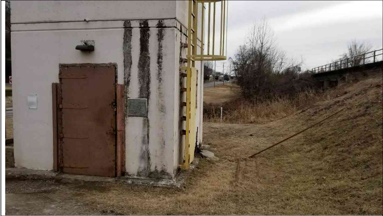
Photo 25 Menard Pumping Station
