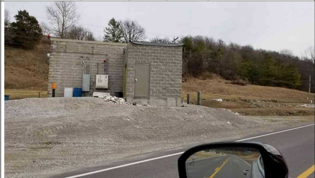
Photo 28 likely the location of the Menard Correctional Center well.
