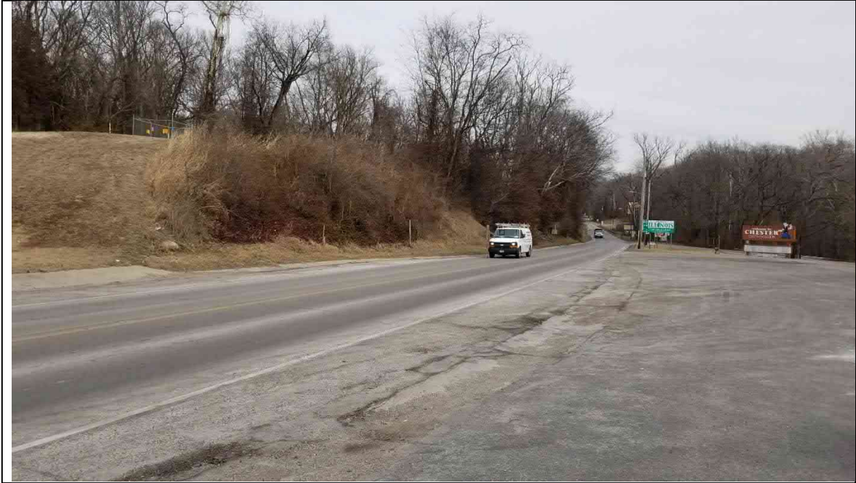
Photo 23, view east of pipeline right of way from bridge
