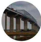
Continuous Through Truss
