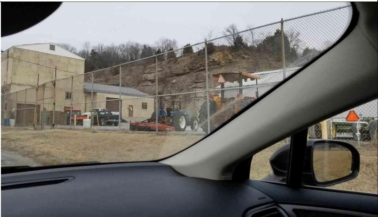
Photo 8 maintenance shop for Menard Correctional
