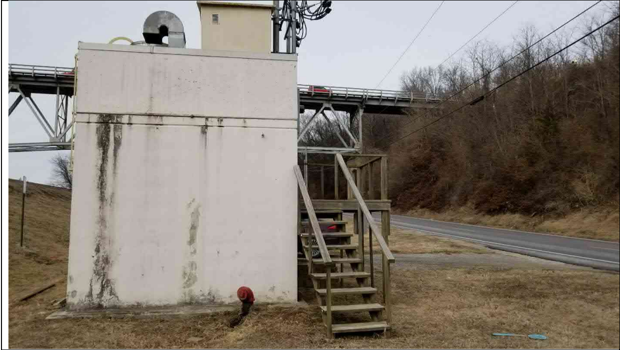
Photo 27 back of pumping station, looking north, bridge in the mid-ground.
