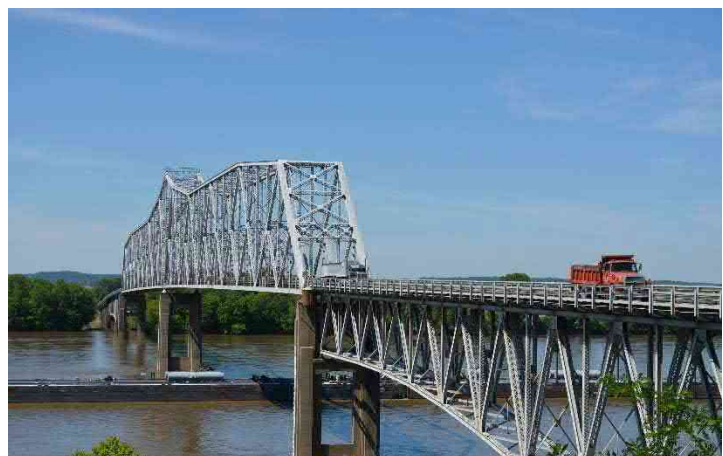
Figure 8 - Typical View from Segar Park
