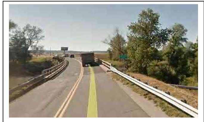
Figure 5 - Typical view of truck crossing center line on curves at the bridge approaches (photo credit: Google Earth).
