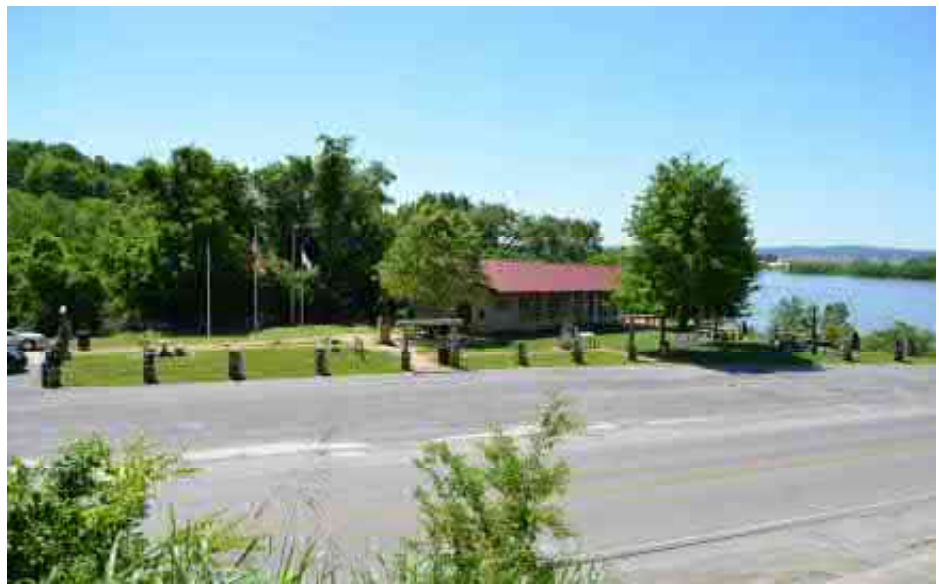
Figure 13 Segar Park with IL Route 150 in Foreground
