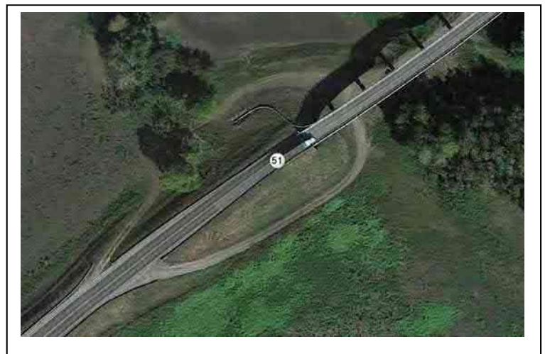
Figure 10 - Typical view of the Route 51 driveways to Horse Island (photo credit: Google Earth).
