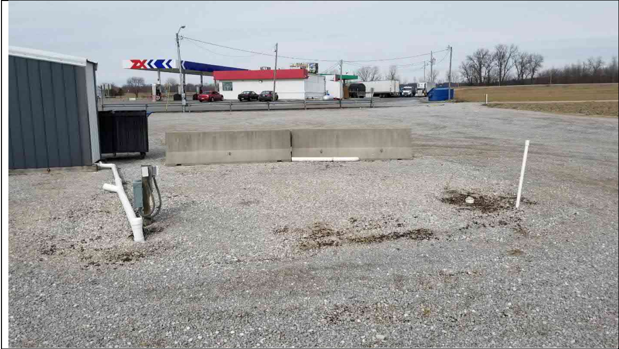
Photo 17 view of likely extraction and injection wells, with the remediation building on left.
