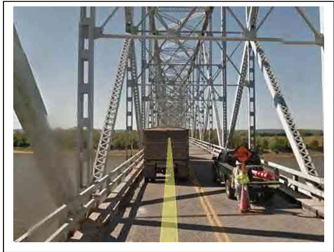
Figure 4 - The Chester Bridge must use lane closures during maintenance or to accommodate over-sized loads (photo credit: Google Earth).
