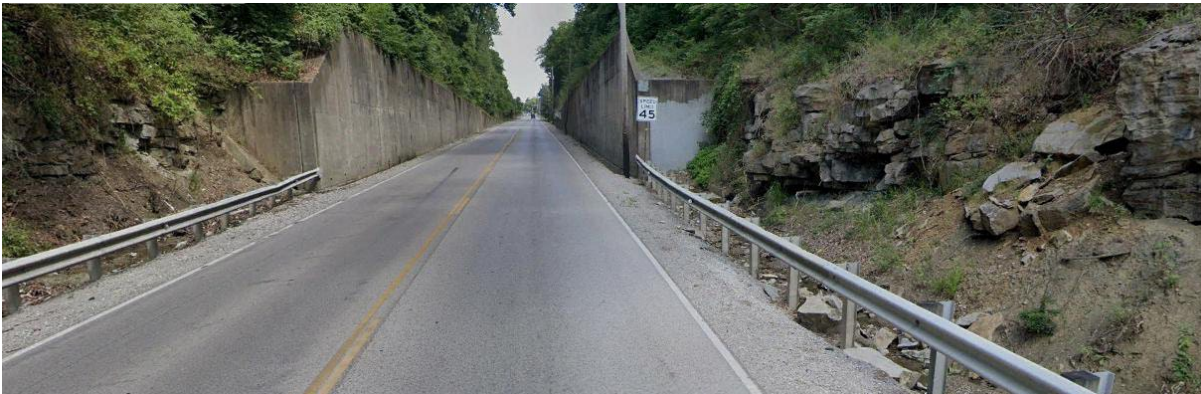
Figure 1-13. View of Route 150/Truck Bypass, North of Valley Street
