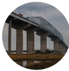
Continuous Through Truss
