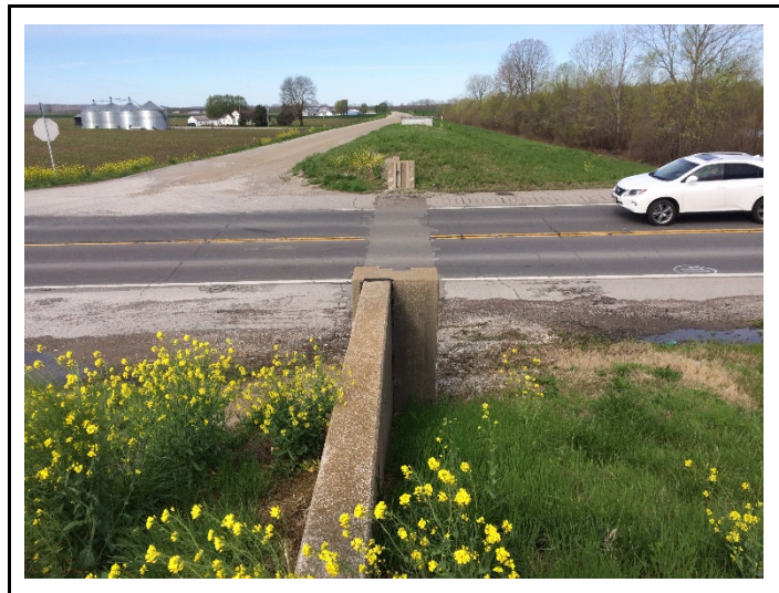
Figure 1-6. Gap in Bois Brule Levee at Route 51
