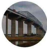
Continuous Through Truss
