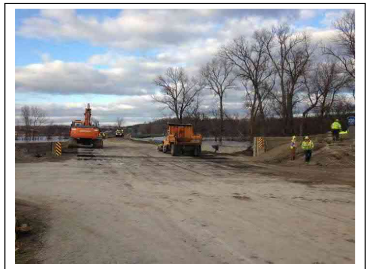
Figure 7 – Heavy equipment is needed to install/remove the Route 51 temporary flood wall.
