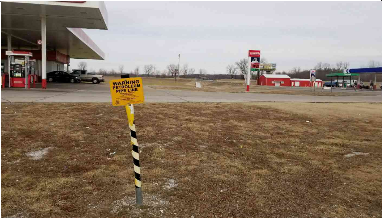
Photo 18 view of Conoco, and location of the buried petroleum pipeline
