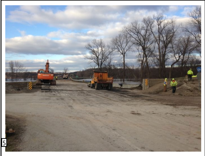
Figure 1-7. Heavy Equipment Used to Install/Remove Route 51 Temporary Flood Wall
