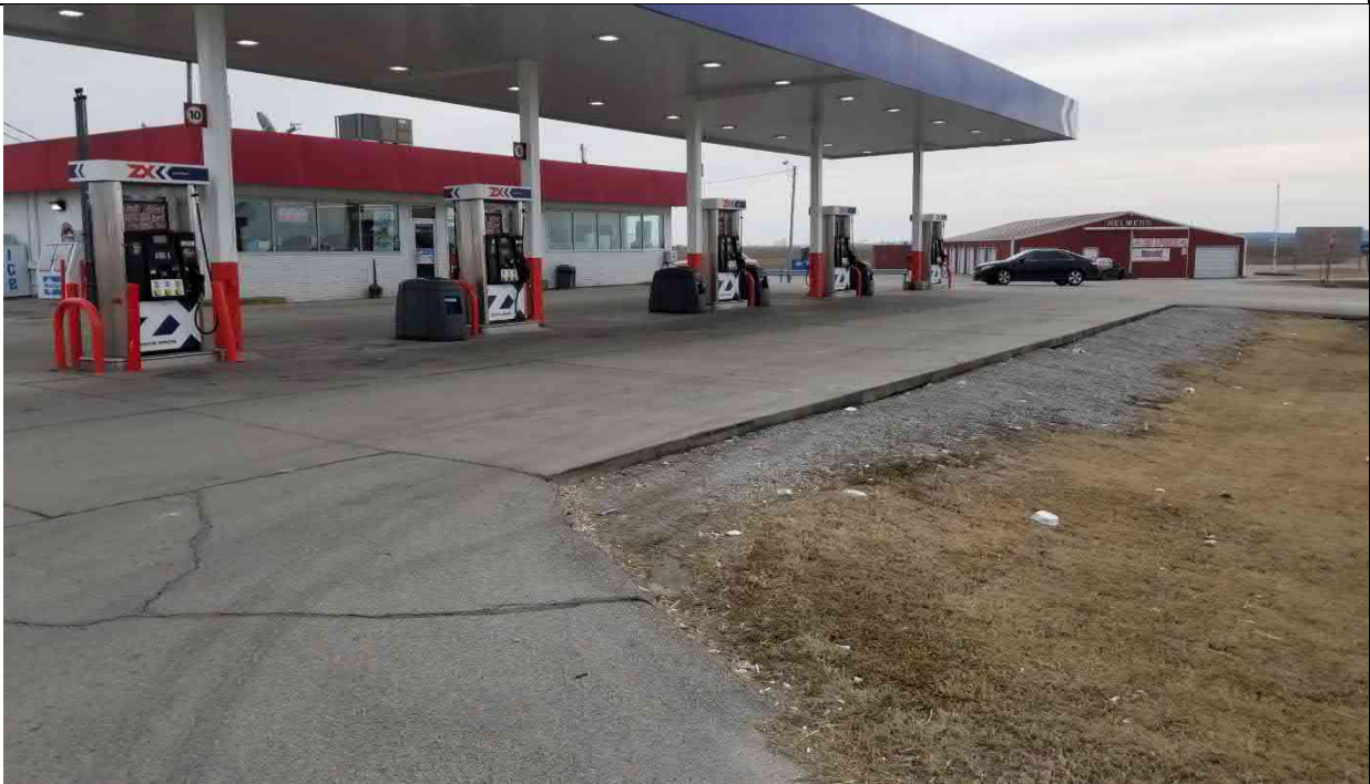
Photo 14 view of the ZX mart gas pumps
