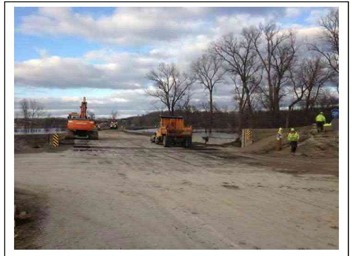
Figure 16 – Heavy equipment is needed to install/remove the Route 51 temporary flood wall.
