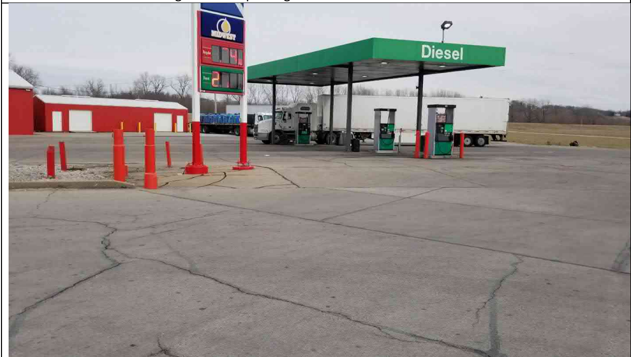
Photo 16 view of diesel pumps at ZX mart
