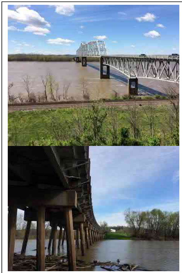
Figure 2 Typical photographs of the Chester Bridge and the Horse Island Chute Bridge
