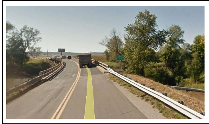
Figure 1-5. Typical View of Truck Crossing Center Line on Curves at the Bridge Approaches (Source: Google Earth)
