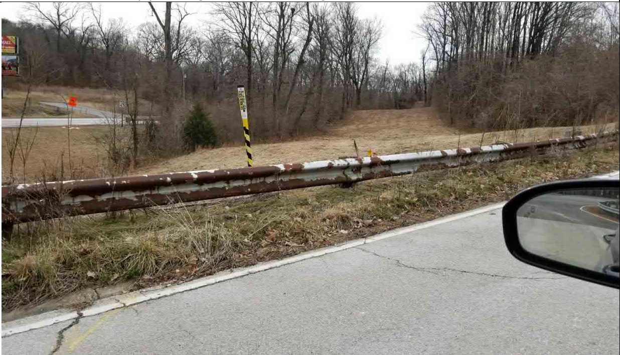
Photo 24 view of pipeline right of way at 200 Rebecca Ln, looking west
