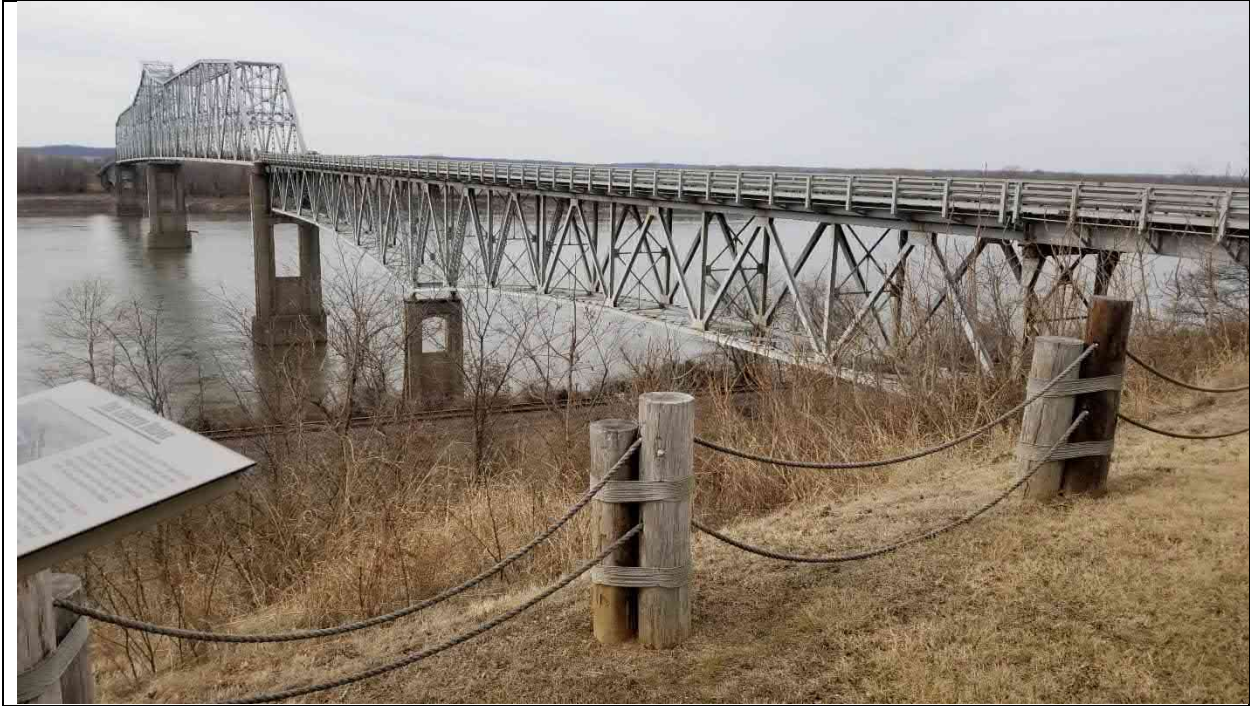
Photo 9, bridge and spill location
