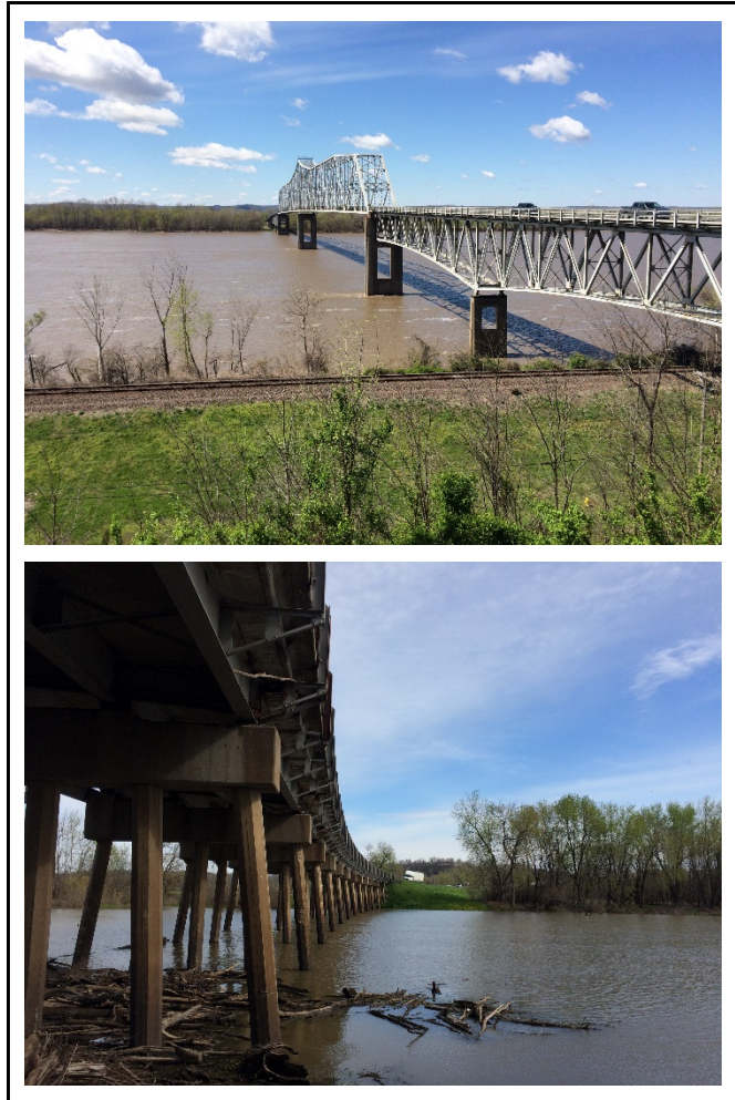
Figure 1-2. Photographs of the Chester Bridge and the Horse Island Chute Bridge
