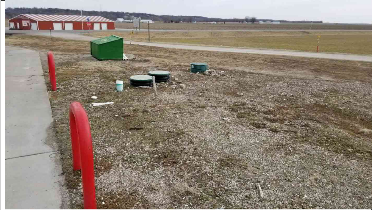
Photo 21 view of likely septic system
