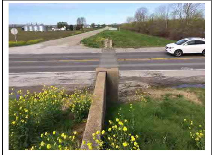
Figure 6 – Gap in Bois Brule levee at Route 51.
