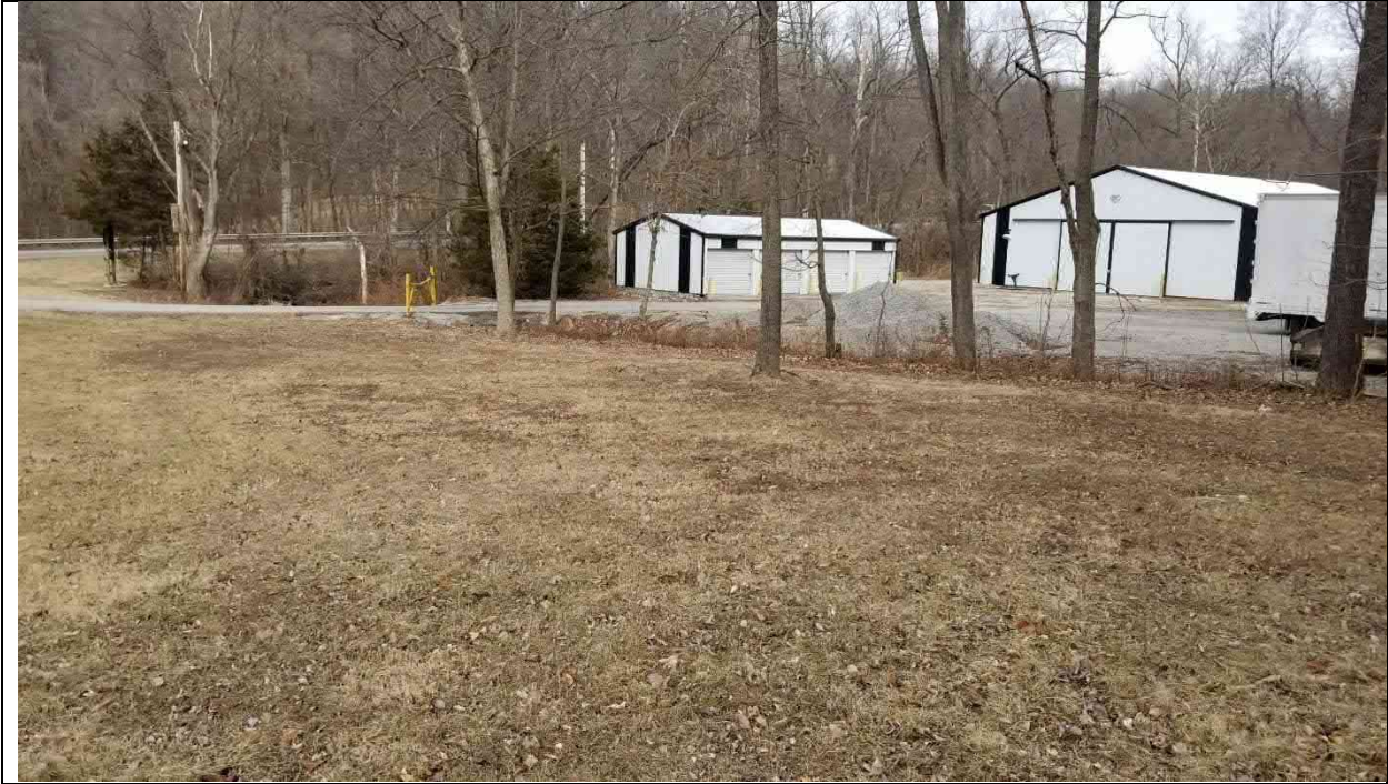
Photo 3 view of Courthouse storage buildings
