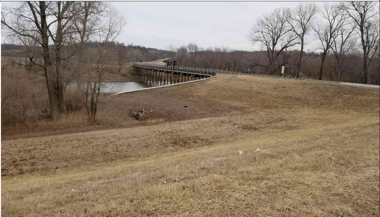
Photo 22 View of pipeline crossing minor channel
