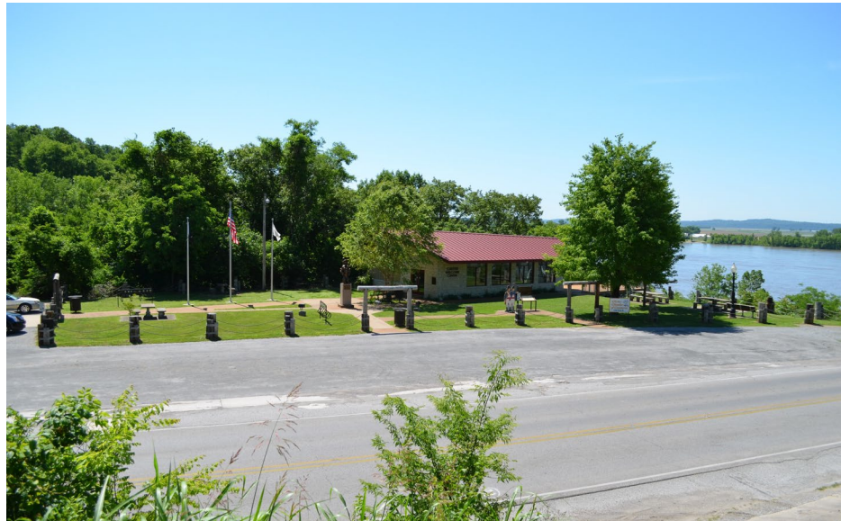
Figure 2-6. Segar Memorial Park with IL Route 150 in Foreground
