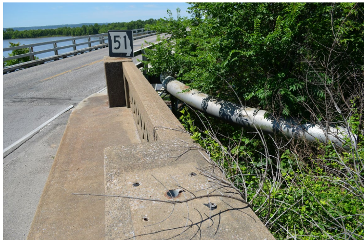
Figure 2-9. Gas Pipeline on Existing Bridge
