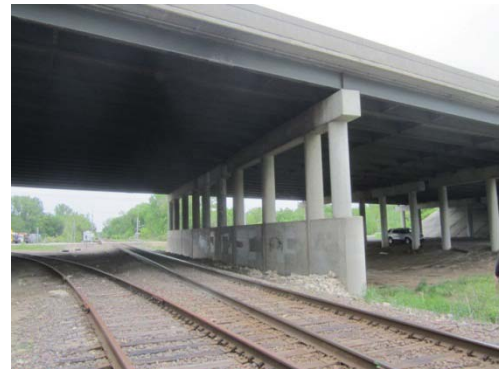
Figure 10. Elevation view looking north
