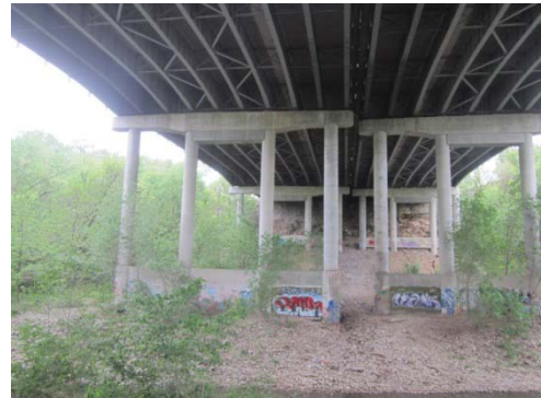
Figure 3. General view of framing and piers
