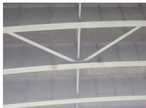
Figure 6. General view of lateral bracing connection
