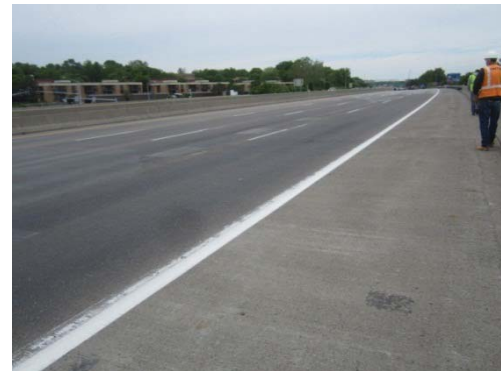
Figure 19. Approach view looking west
