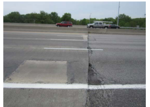
Figure 13. Deck patching at abutment
