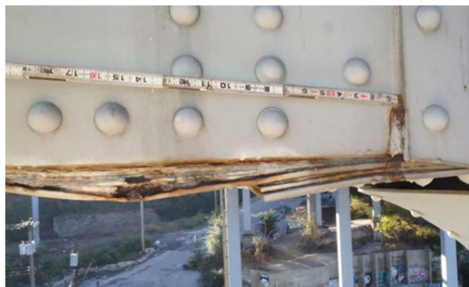
Figure 8: Corrosion at approach piers
