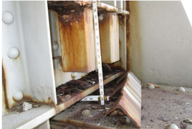
Figure 4: Broken retainer angle at suspender cable socket
