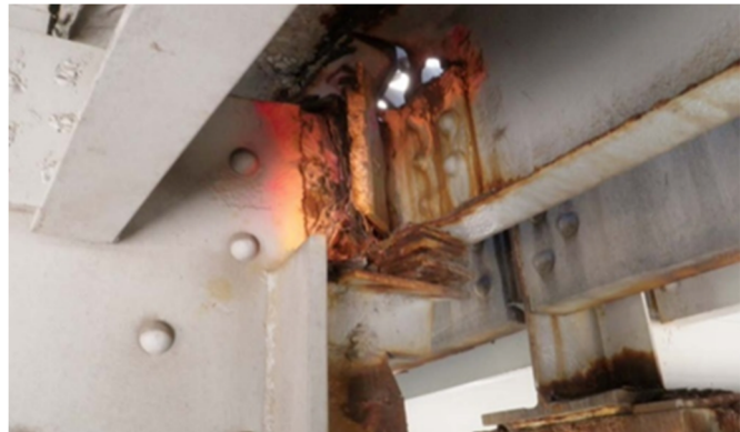
Figure 5: Deterioration at expansion joint support
