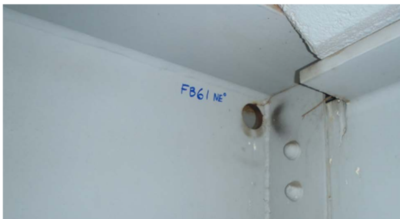
Figure 10: Fatigue cracking in southbound north approach spans
