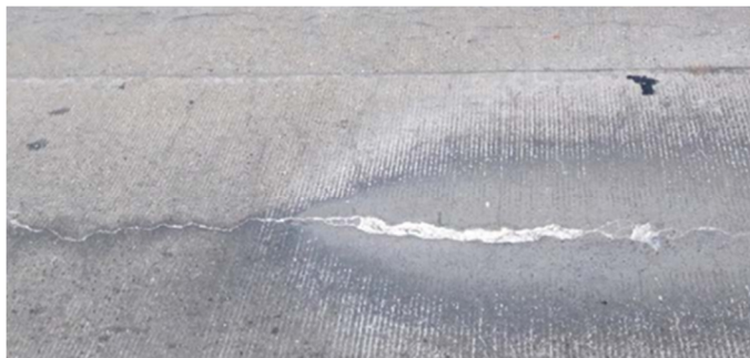
Figure 6: Deck cracking in overlay (left), corrosion and spalling at railing parapets (right)
