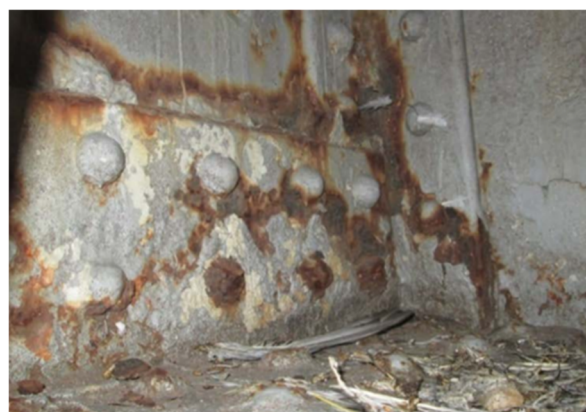
Figure 3: Typical deterioration at steel elements
