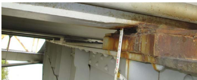
Figure 2: Pack rust at stringer bearing plates
