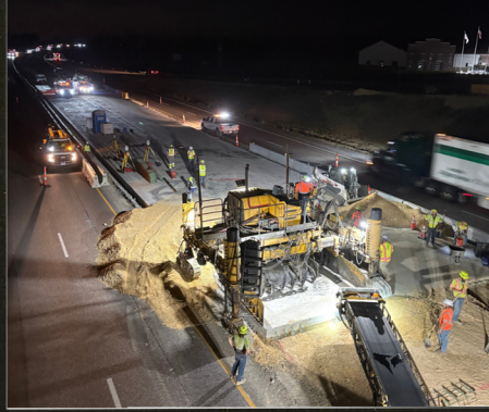
I-70 pavement work between Columbia and Kingdom City.
