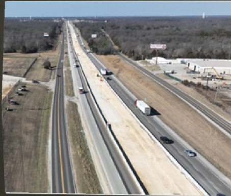
Paving progress between Warrenton and Wentzville.
