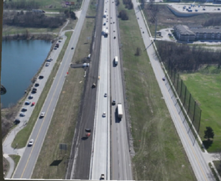
I-70 pavement progress between Blue Springs and Odessa.
