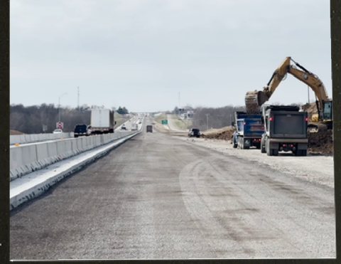
New westbound I-70 pavement construction.
