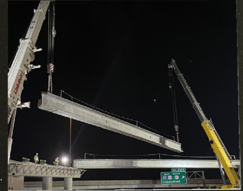
Bridge girder work along southbound U.S. 61 over I-70.
