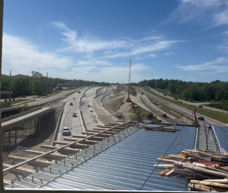
Future northbound U.S. Route 63 fly over ramp to westbound I-70.
