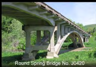
Round Spring Bridge No. J0420
