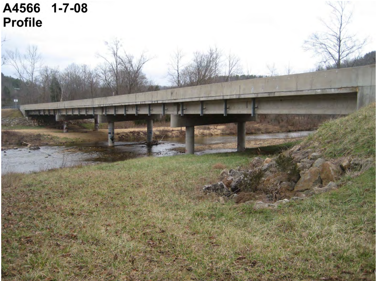
P/S I Girder Bridge Example
