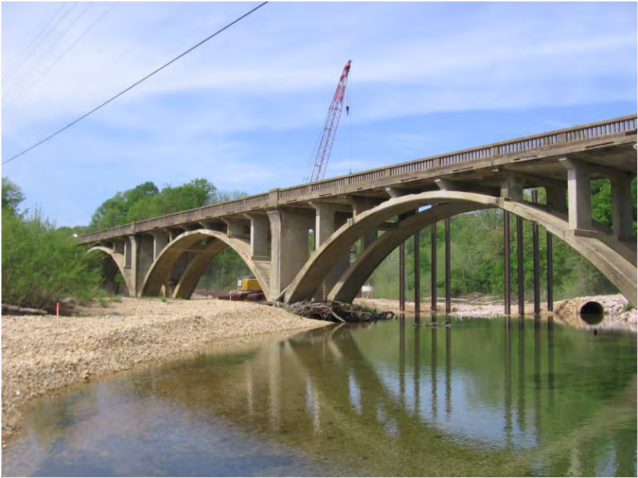
Sinking Creek Bridge (H0079), facing southwest
