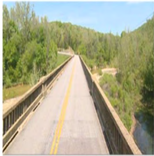
On the bridge, looking north
