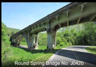
Round Spring Bridge No. J0420
