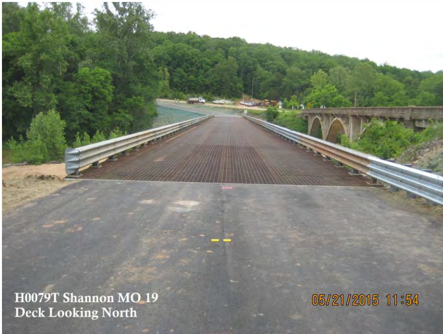
Sinking Creek Temporary Bridge (H0079T), facing north
