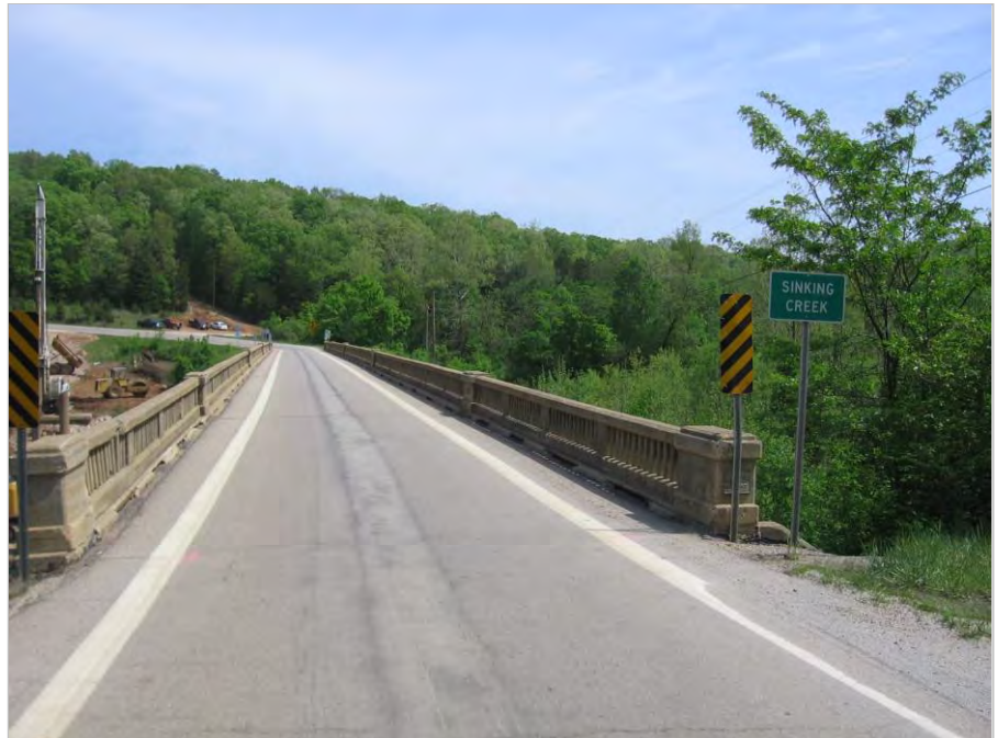
Shannon County Route 19 MoDOT Job No. J9P0438
