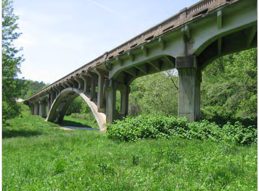
Shannon County Route 19 MoDOT Job No. J9P0438
