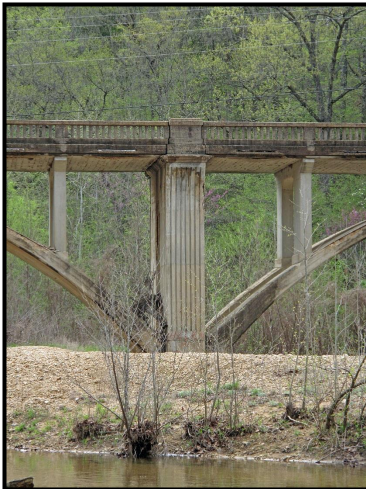
Figure 12: Sinking Creek Bridge, facing east, Column detail
