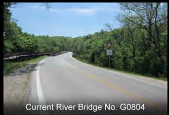
Current River Bridge No. G0804
