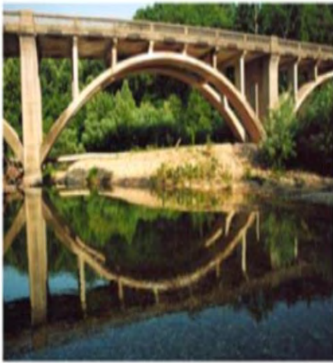
MO Route 19 Sinking Creek Bridge, Looking southeast
