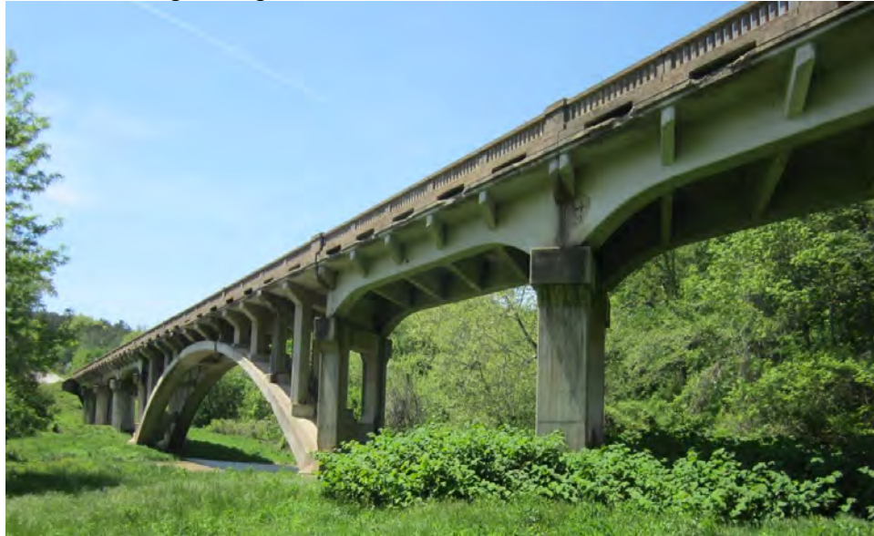
Figure 4: Spring Valley Bridge (2015)
