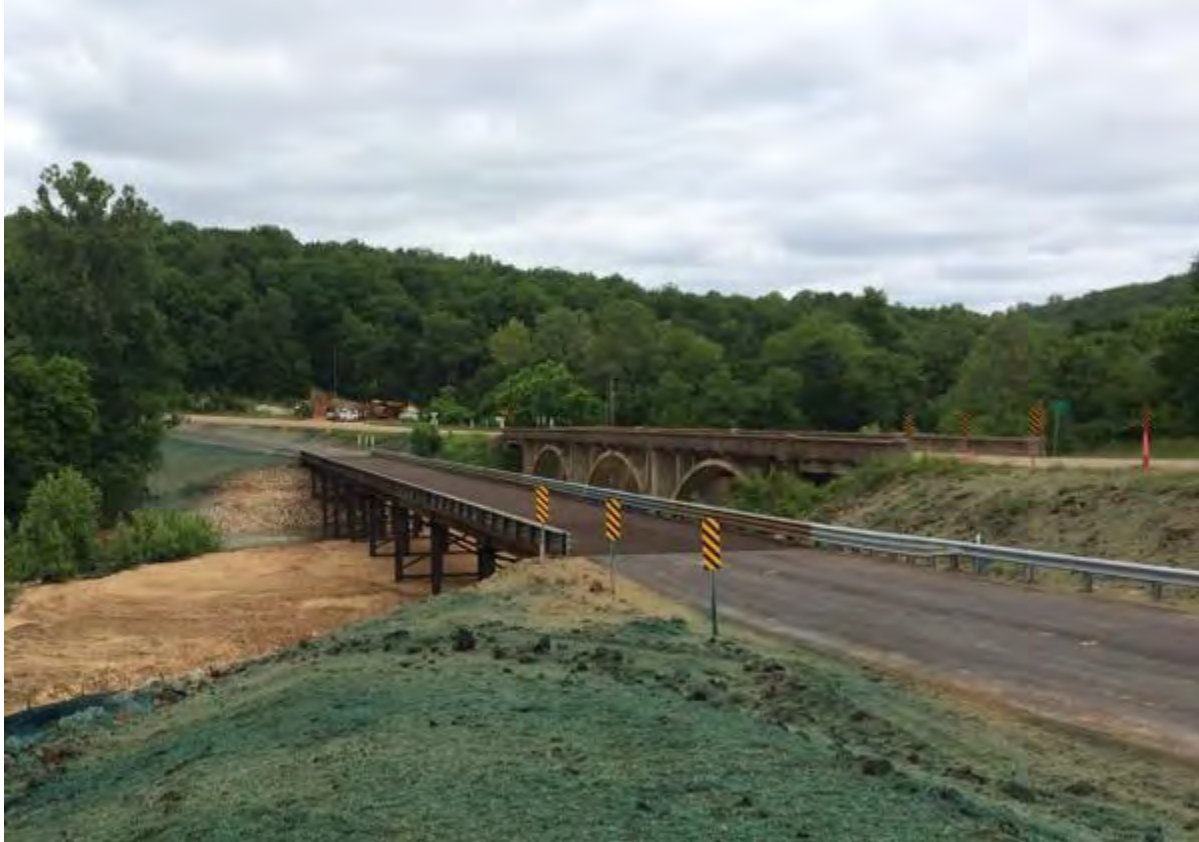
Figure 1-5: Temporary Bridge Photo
