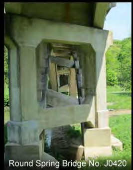
Round Spring Bridge No. J0420
