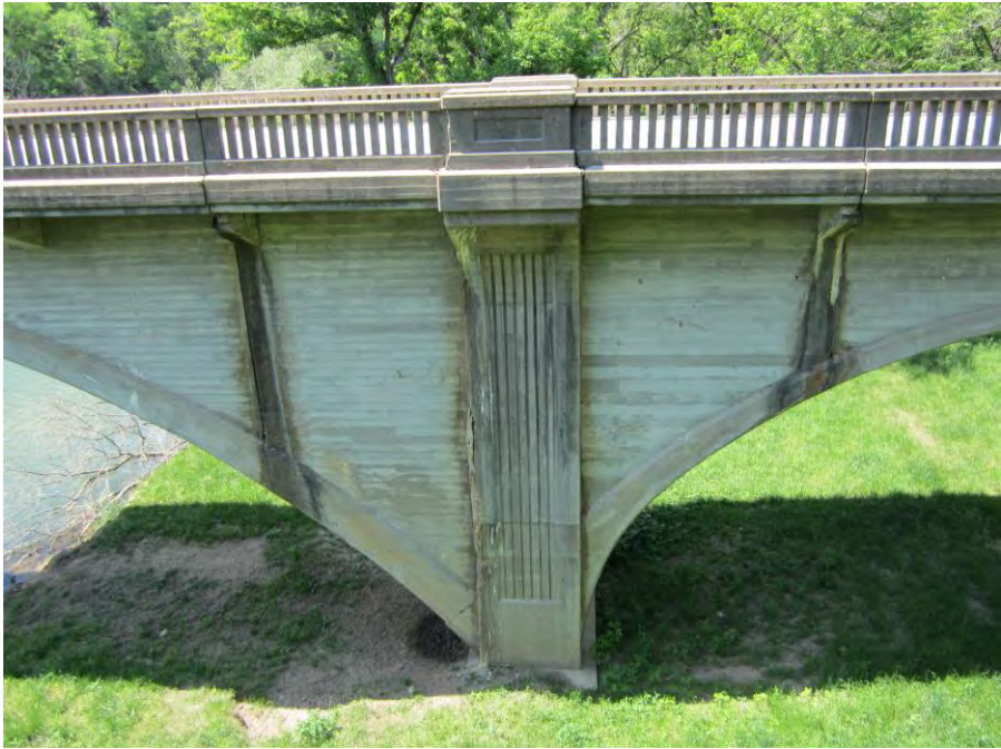
Current River Bridge (G0804), facing east
