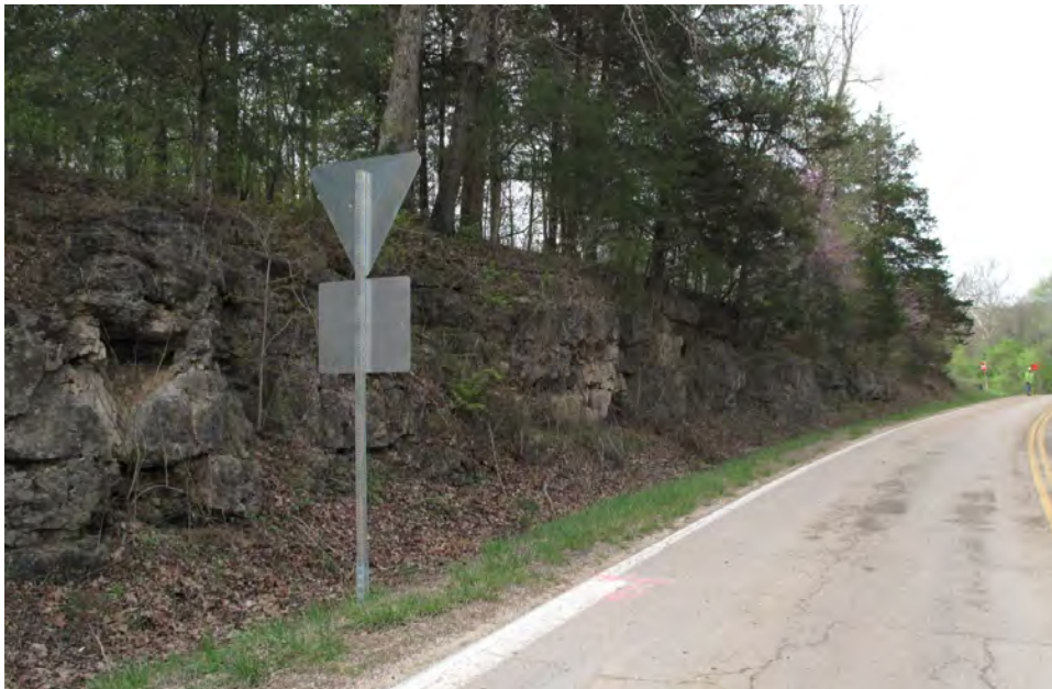
Figure 5: Representative example of rock cuts along Route 19 near Sinking Creek (2015)
