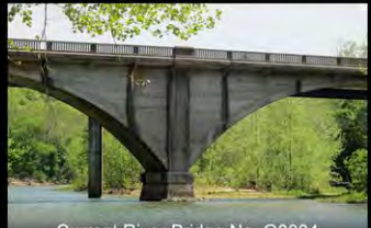
Current River Bridge No. G0804
