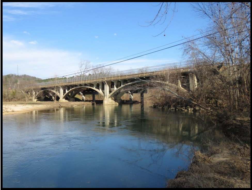
Figure 19: Eminence Bridge, side view
