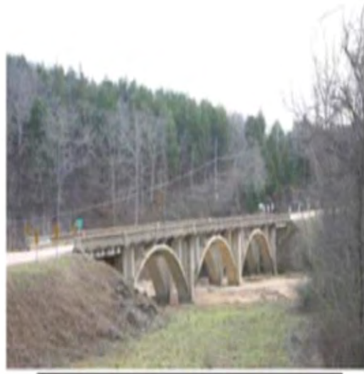
South bound on MO 19, looking at west side of bridge
