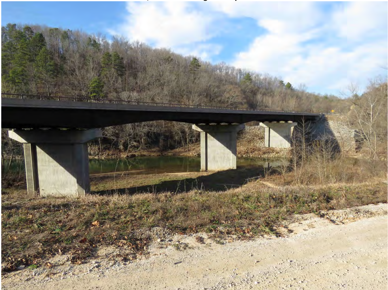
Haunched Plate Girder Bridge Example
