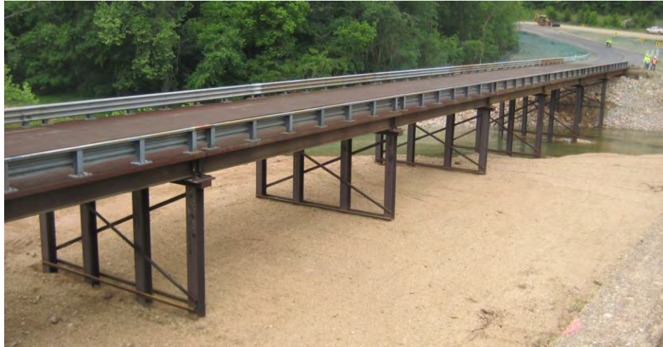
Figure 2: Temporary Bridge at Sinking Creek (2015)
