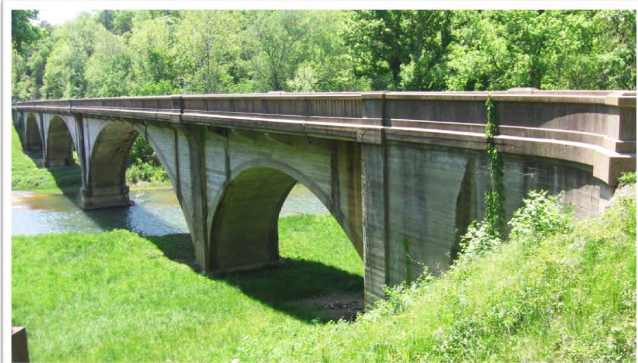
Figure 6: Current River Bridge (G0804)
