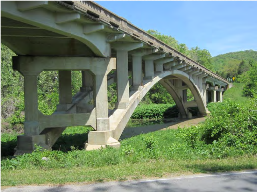
Spring Valley (Round Spring) Bridge (J0420), facing northwest
