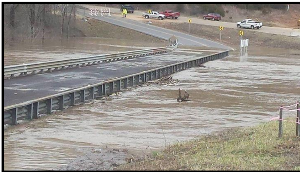
Figure 4: Temporary Bridge closed due to flooding
