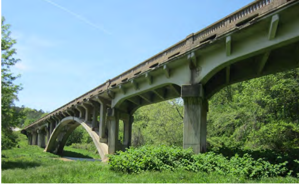
Figure 4: Spring Valley Bridge (2015)
