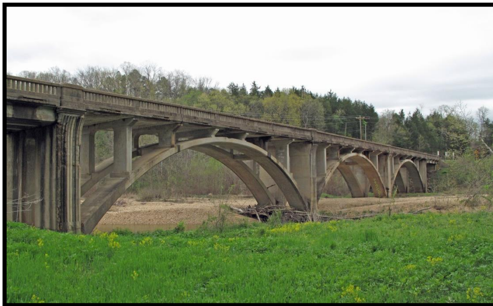
Figure 11: Sinking Creek Bridge, facing southeast
