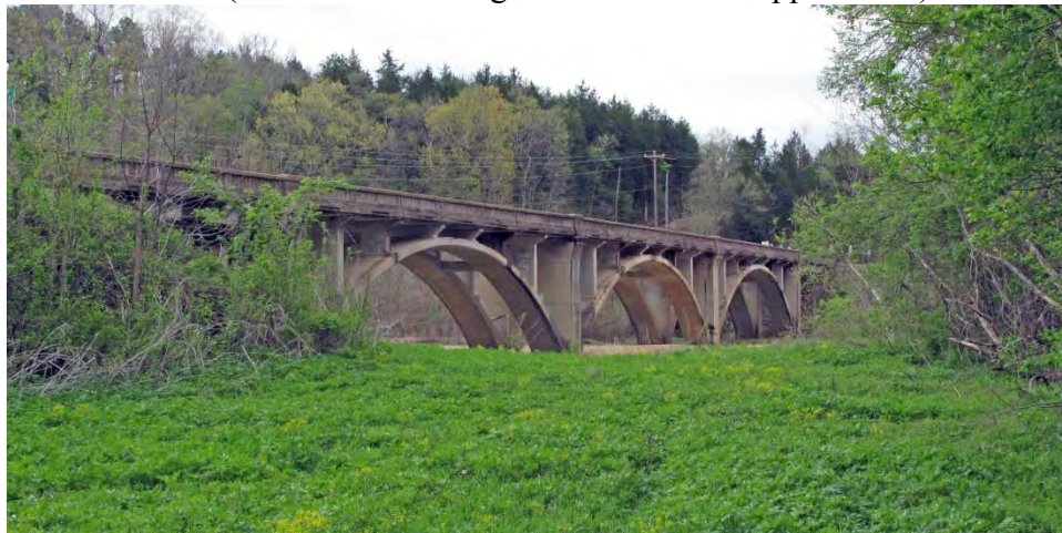
Figure 1: Sinking Creek Bridge (2015)
