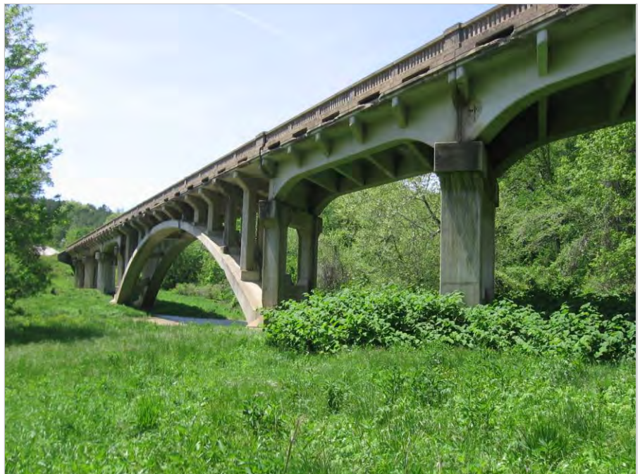
Shannon County Route 19 MoDOT Job No. J9P0438
