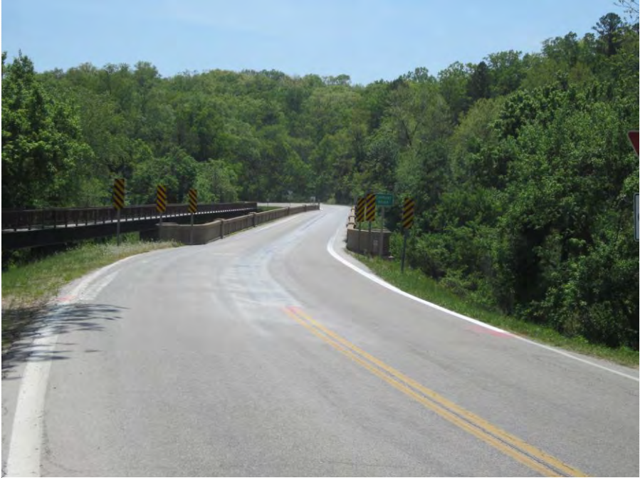
Current River Bridge (G0804), facing south
