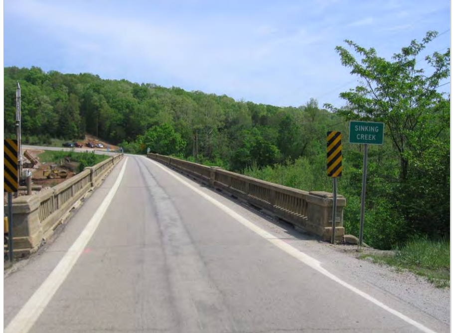
Shannon County Route 19 MoDOT Job No. J9P0438
