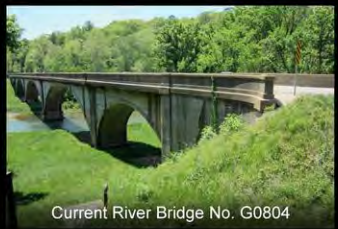
Current River Bridge No. G0804
