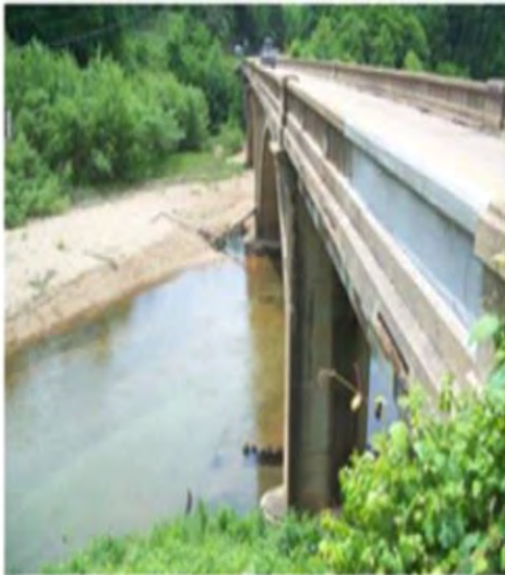
East side of bridge, South approach
