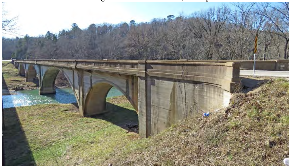
Figure 3: Current River Bridge (2015)
