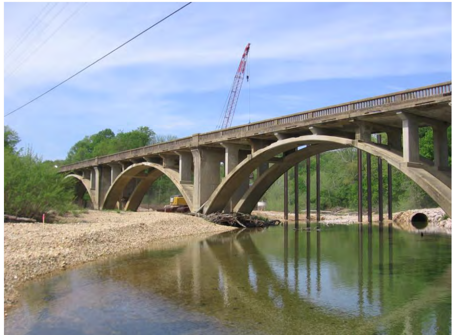
Sinking Creek Bridge (H0079), facing southwest
