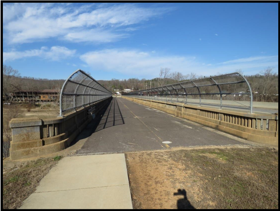
Figure 18: Eminence Bridge, deck view
