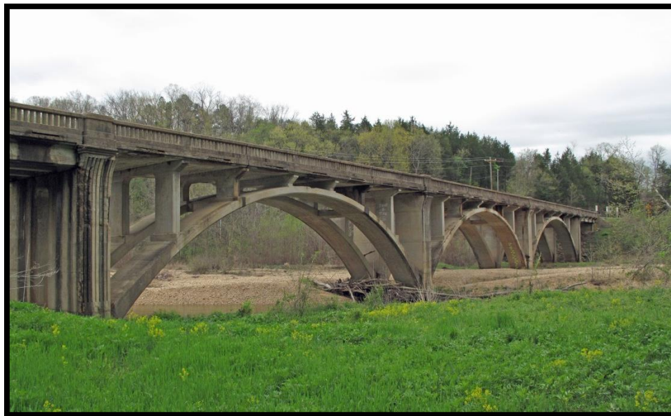
Figure 11: Sinking Creek Bridge, facing southeast
