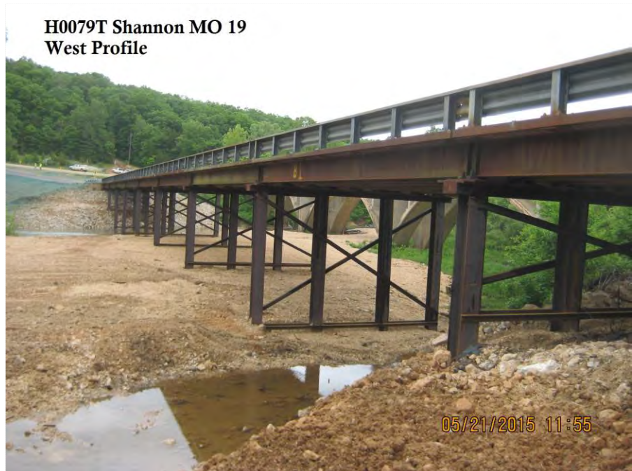
Sinking Creek Temporary Bridge (H0079T), facing north
