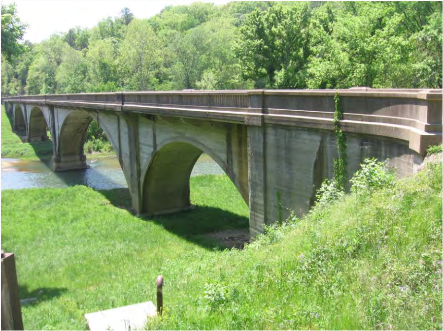
Current River Bridge (G0804), facing northwest
