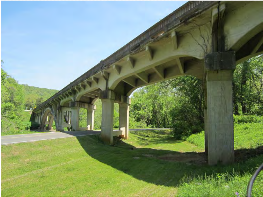
Spring Valley (Round Spring) Bridge (J0420), facing northeast
