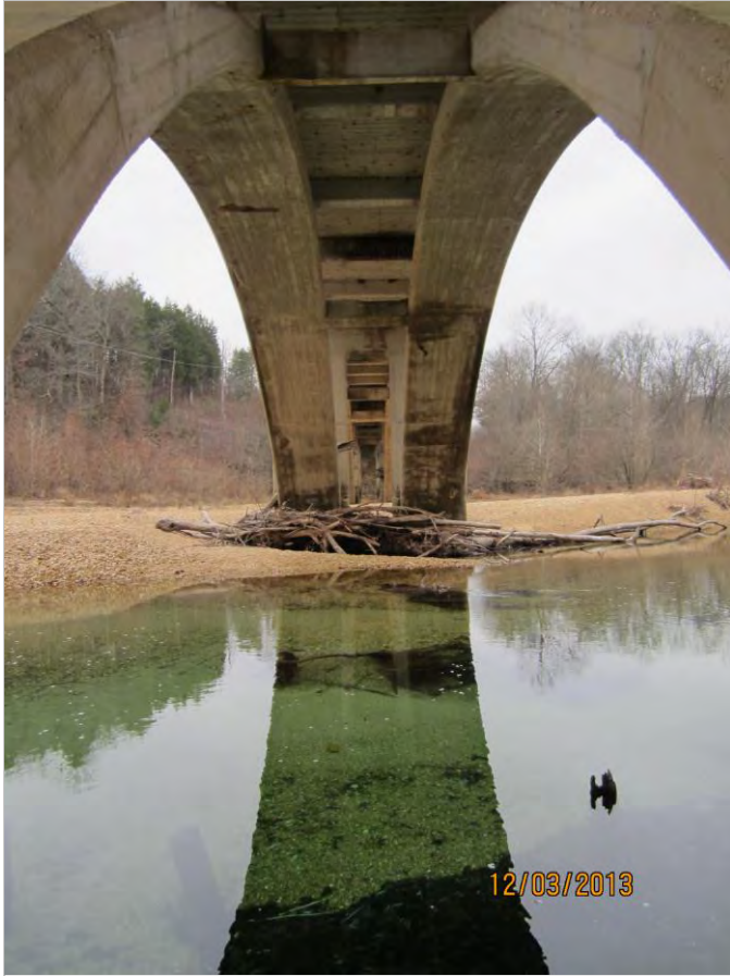
Sinking Creek Bridge (H0079), facing south
