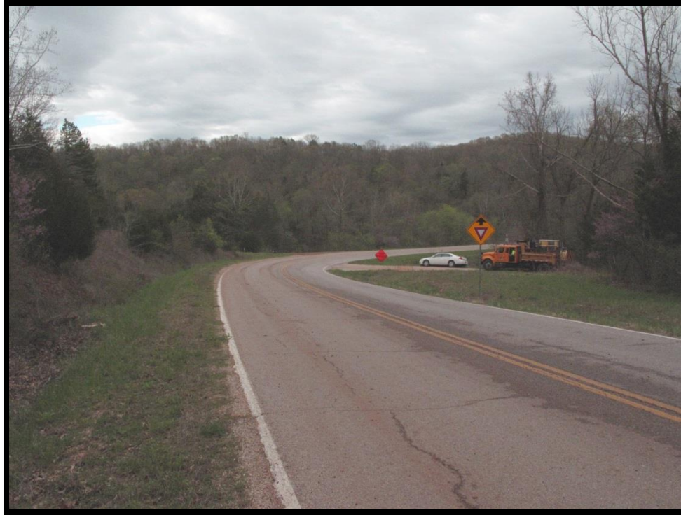
Figure 15: Three Bridges Historic District, view leading into Sinking Creek Bridge
