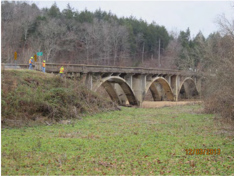
Sinking Creek Bridge (H0079), facing southeast
