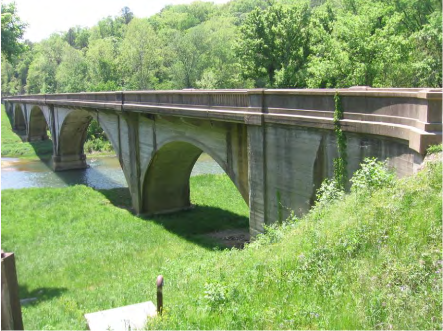
Current River Bridge (G0804), facing northwest
