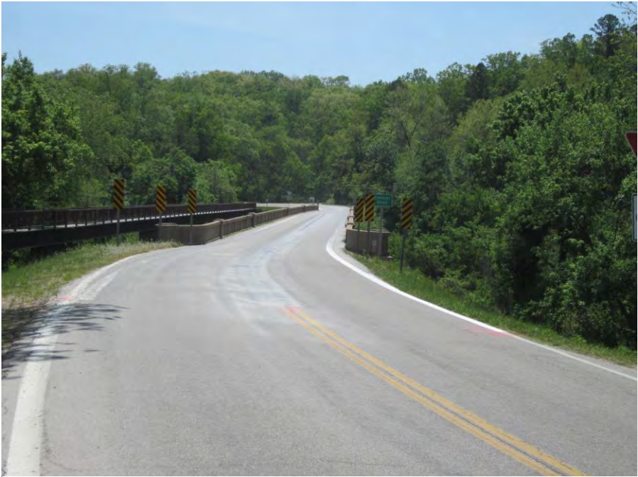
Current River Bridge (G0804), facing south
