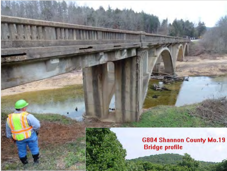
Sinking Creek Bridge, H0079
