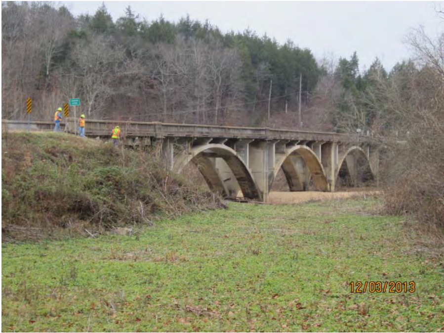
Sinking Creek Bridge (H0079), facing southeast
