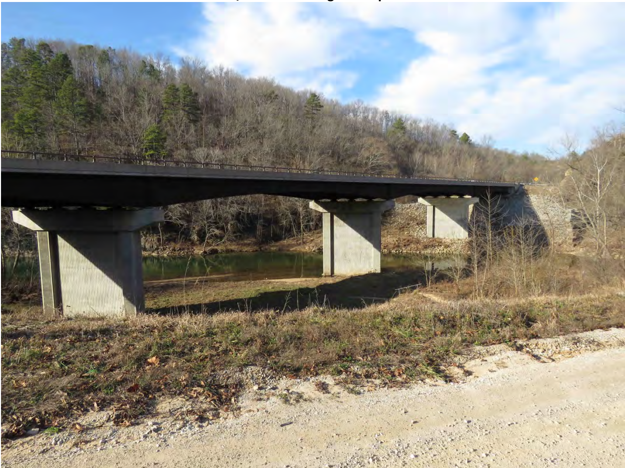
Haunched Plate Girder Bridge Example
