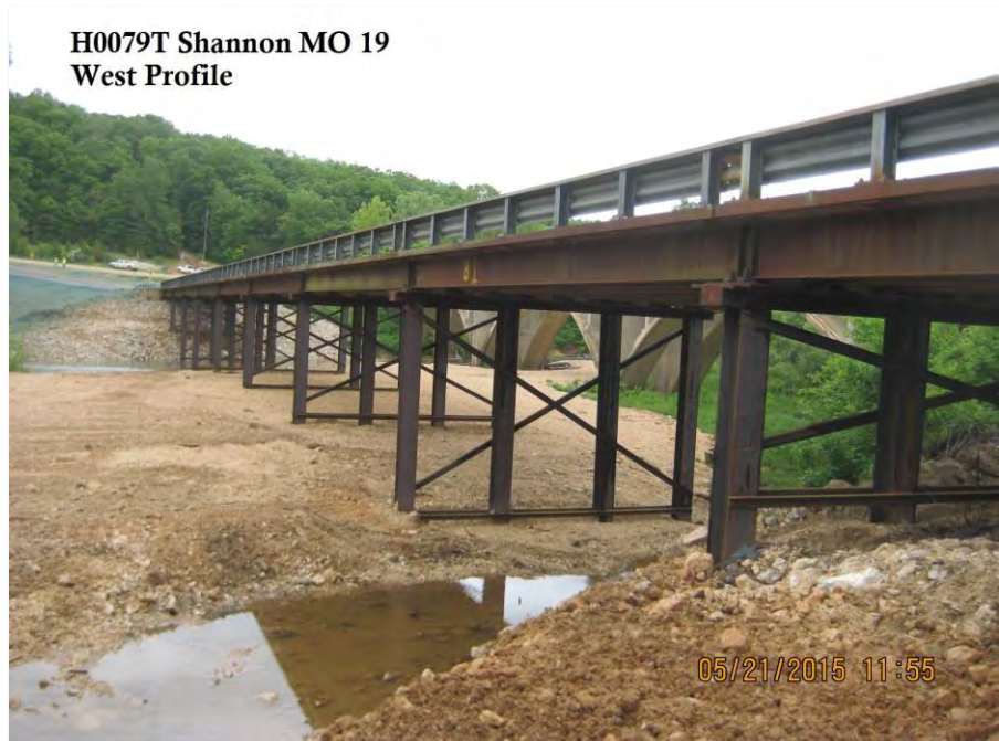
Sinking Creek Temporary Bridge (H0079T), facing north
