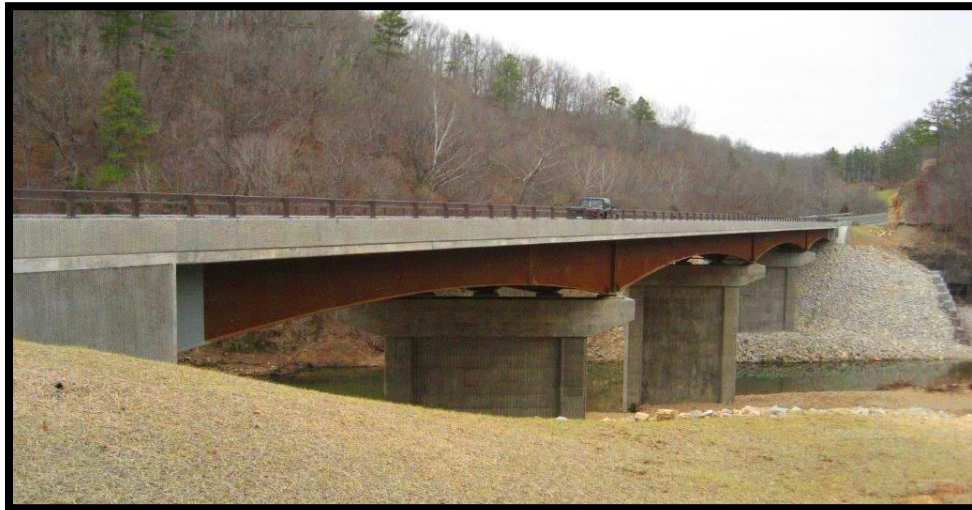
Figure 20: Example of a Haunched Plate Girder: Buck Hollow Bridge, Texas County
