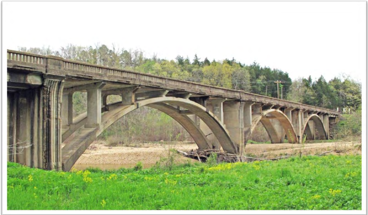
Figure 5: Sinking Creek Bridge (H0079)
