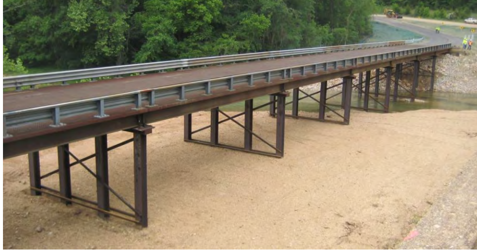
Figure 2: Temporary Bridge at Sinking Creek (2015)
