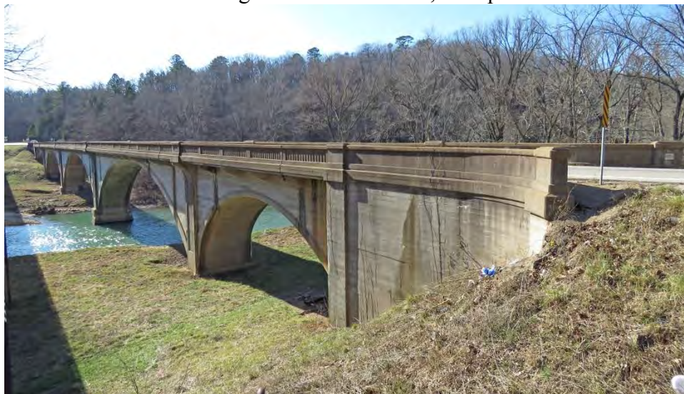
Figure 3: Current River Bridge (2015)
