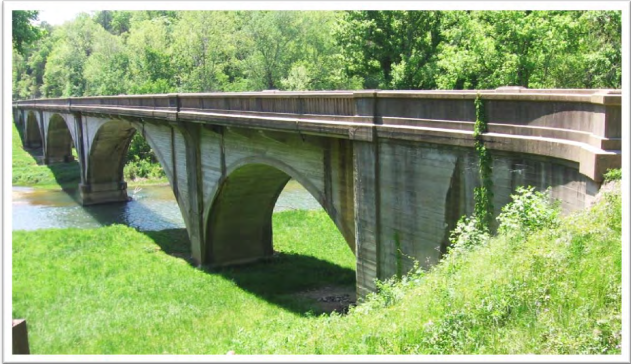
Figure 6: Current River Bridge (G0804)
