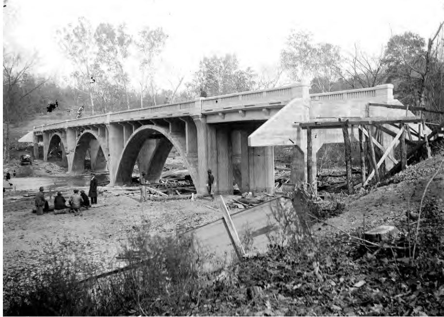
Figure 12: Sinking Creek Bridge during construction, (Gill 1926)
