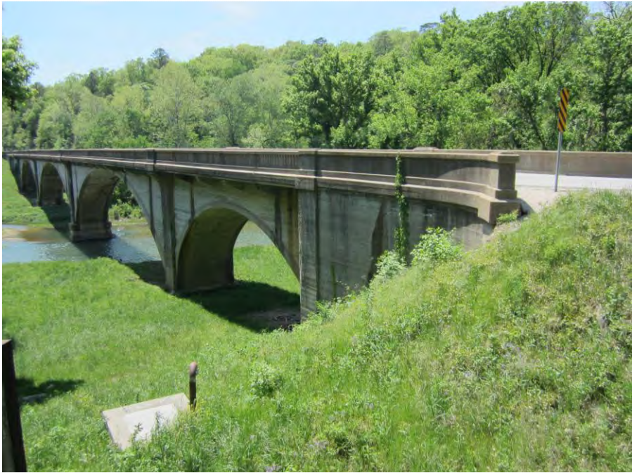
Current River Bridge (G0804), facing southwest
