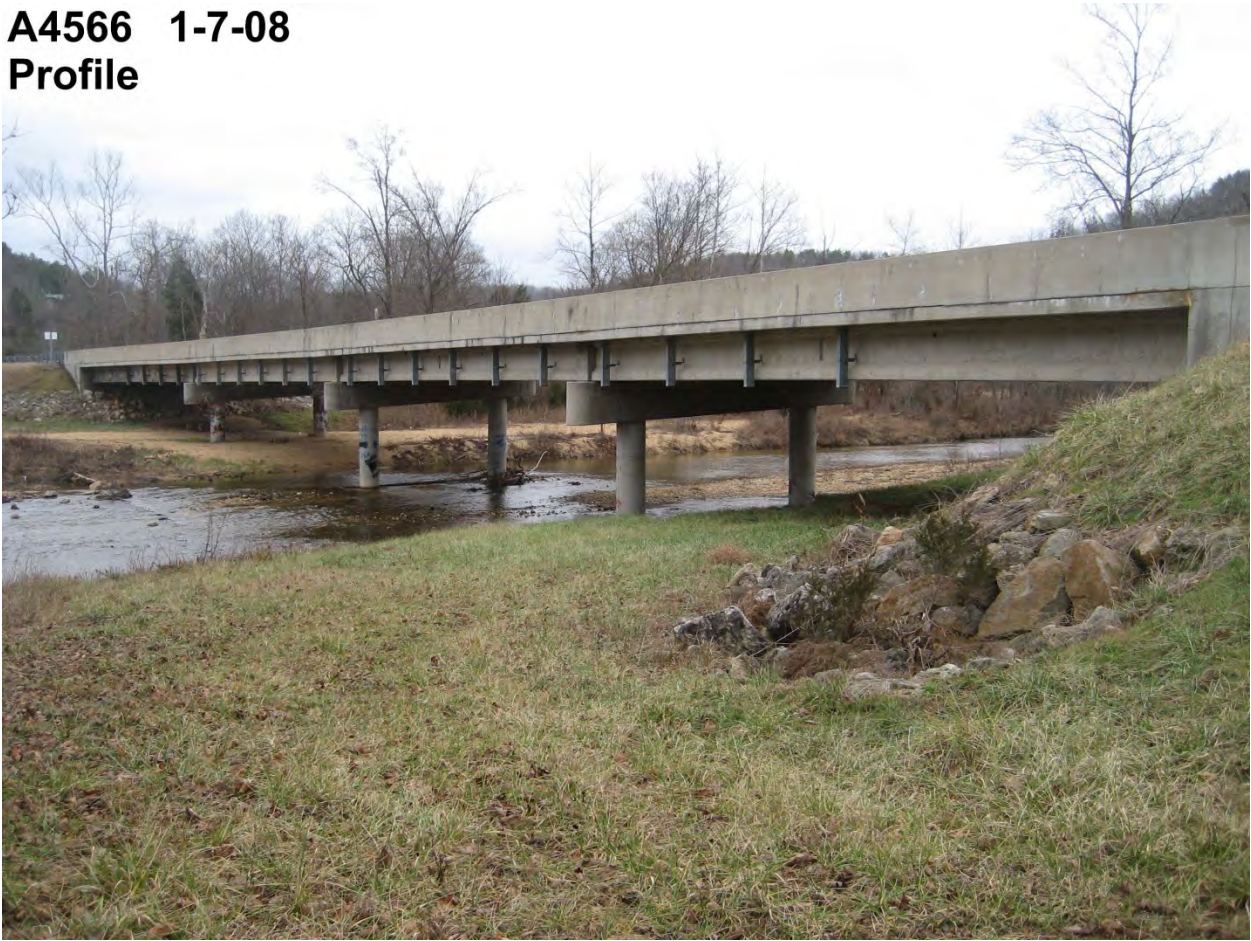
P/S I Girder Bridge Example
