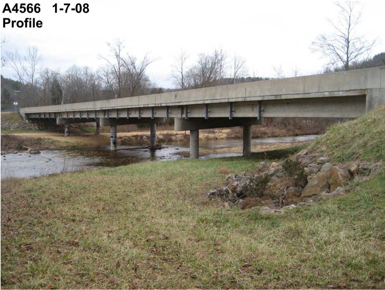
P/S I Girder Bridge Example
