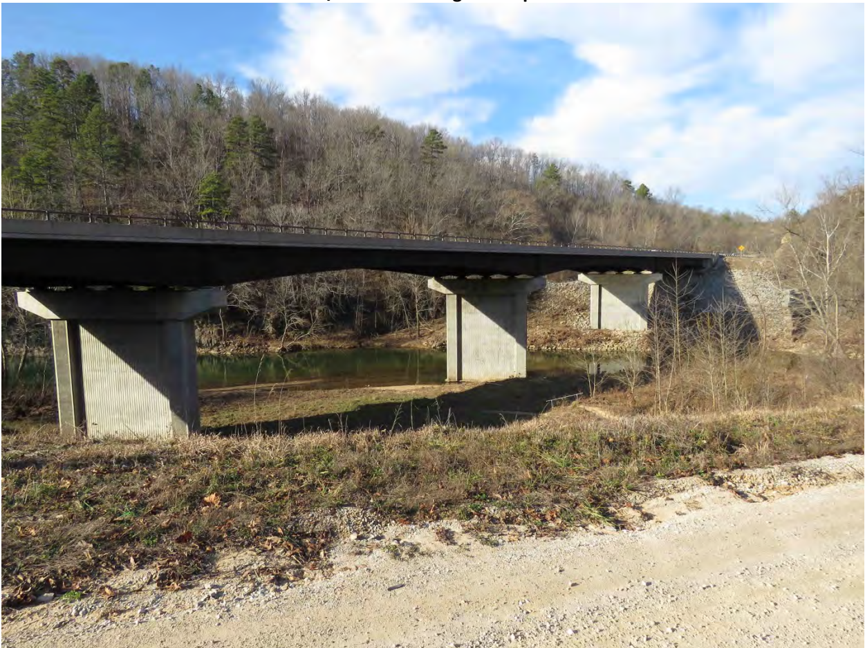
Haunched Plate Girder Bridge Example
