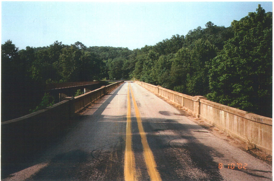
Roadway - Looking South (Note utility/pedestrian bridge at left)
