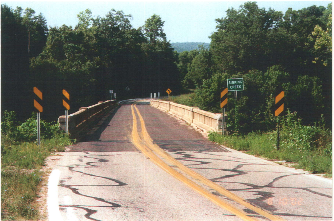
Roadway - Looking South
