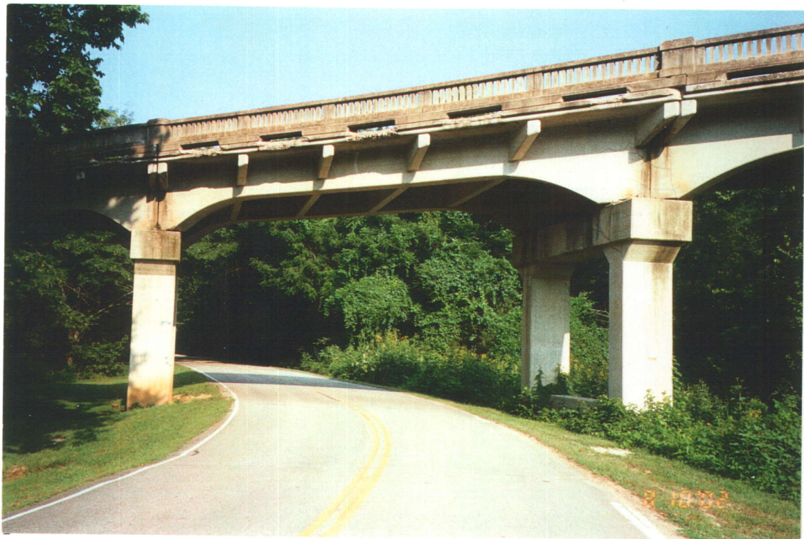
Span Over Park Road - Looking East
