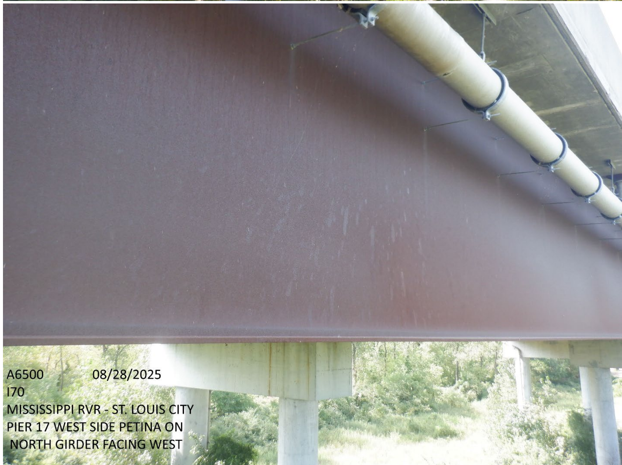
A6500 08/28/2025 170 MISSISSIPPI RVR - ST. LOUIS CITY PETINA BOTTOM OF WEB PIER 17
