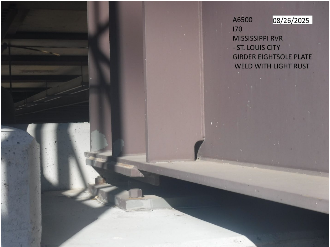
A6500 10/25/2025 I70 MISSISSIPPI RVR - ST. LOUIS CITY GIRDER SIX COLUMN DAMAGE @ BOTTOM OF GIRDER
