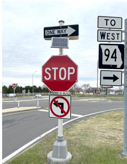
Figure 11: LED stop sign with a solar charger
