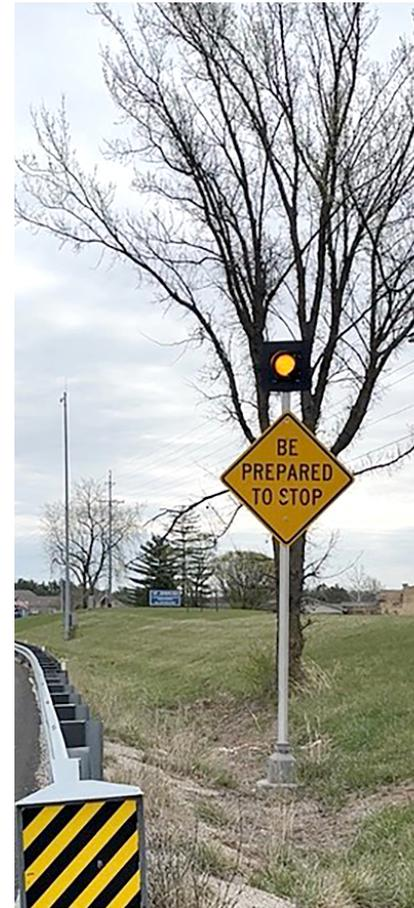
Figure 14: Flashing beacon on top of a warning sign
