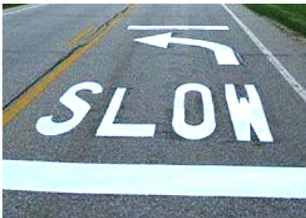
Figure 13: Curve warning pavement marking
