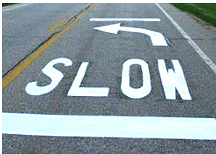
Figure 13: Curve warning pavement marking
