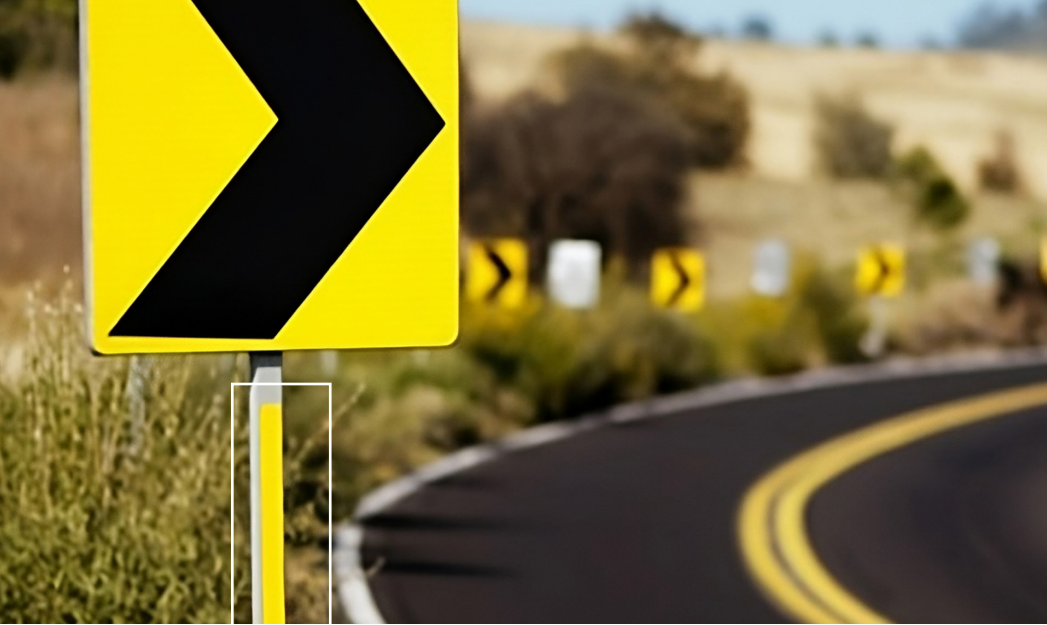
Figure 15: Chevrons with reflective signpost strip
