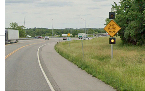
Figure 9: Intersection conflict warning system
