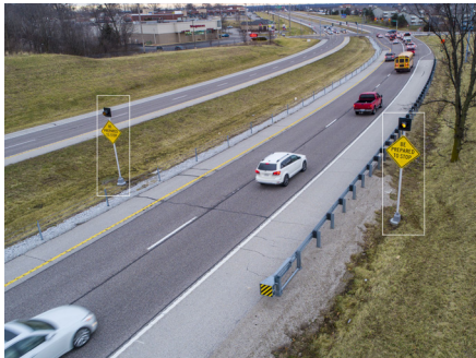
Figure 12: Dynamic signal warning flashers
