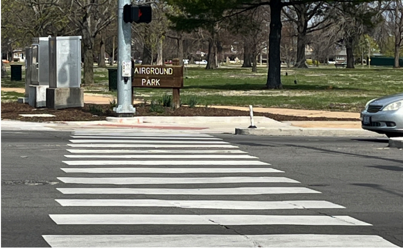
Figure 26: High visibility crosswalk
