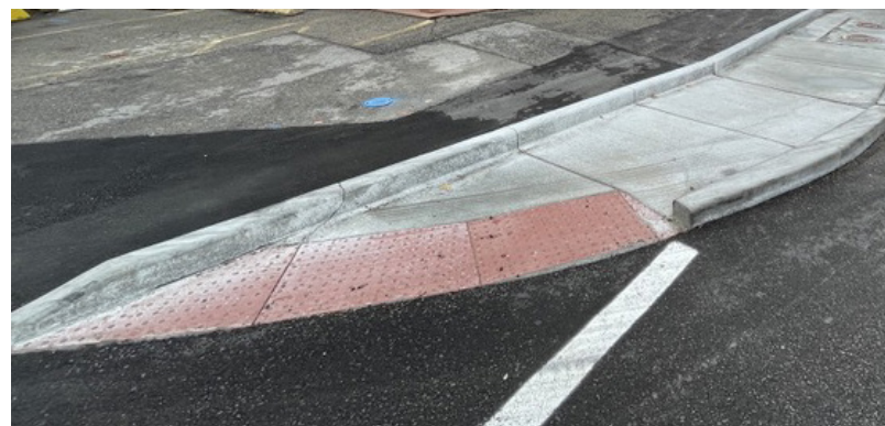
Figure 25: ADA curb ramp
