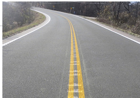
Figure 8: Centerline rumble strip
