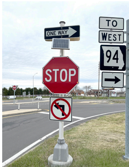
Figure 11: LED stop sign with a solar charger
