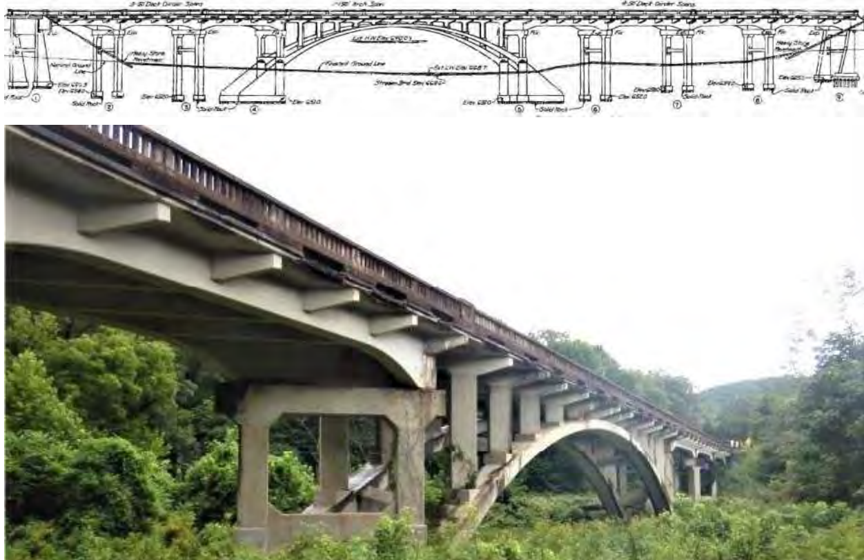
Figure 3: Spring Valley Creek Bridge Diagram and Photograph (J0420)
