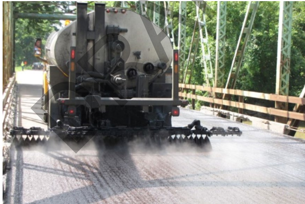
Typical bridge sealing
