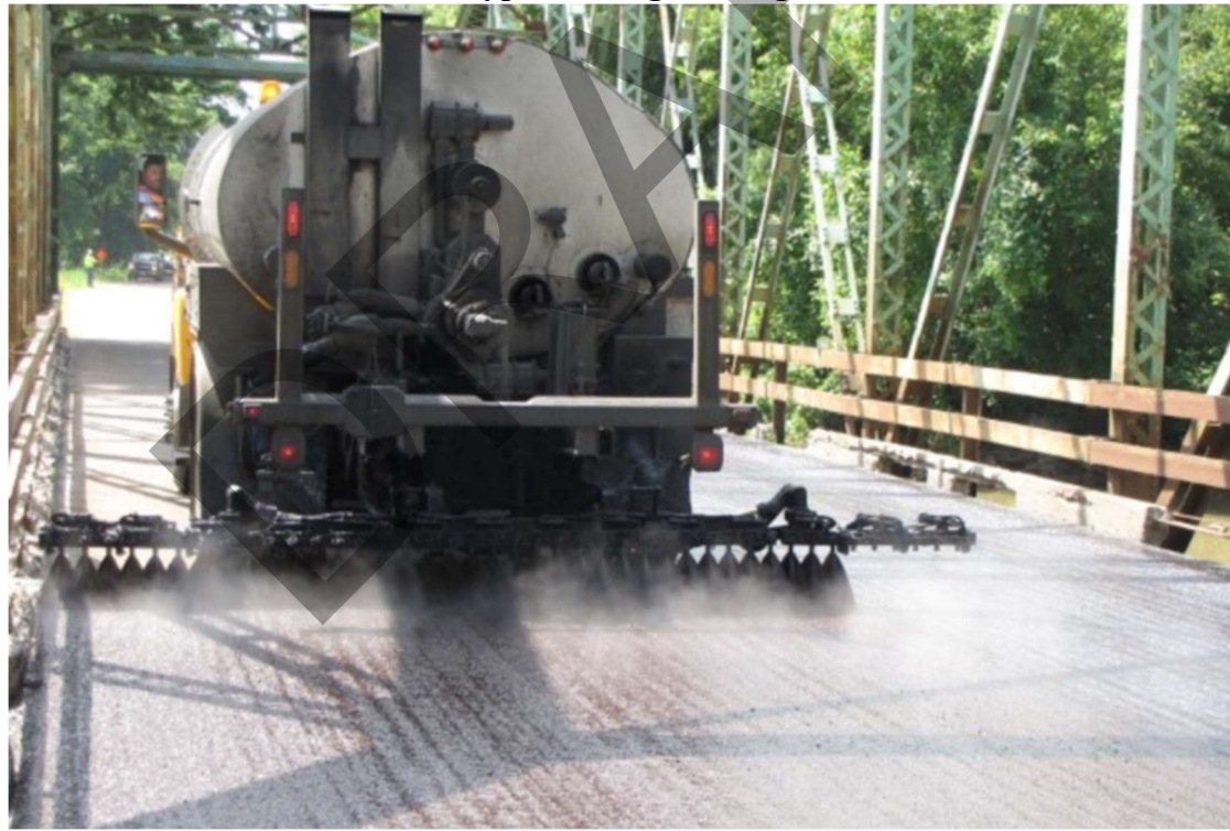
Typical bridge sealing
