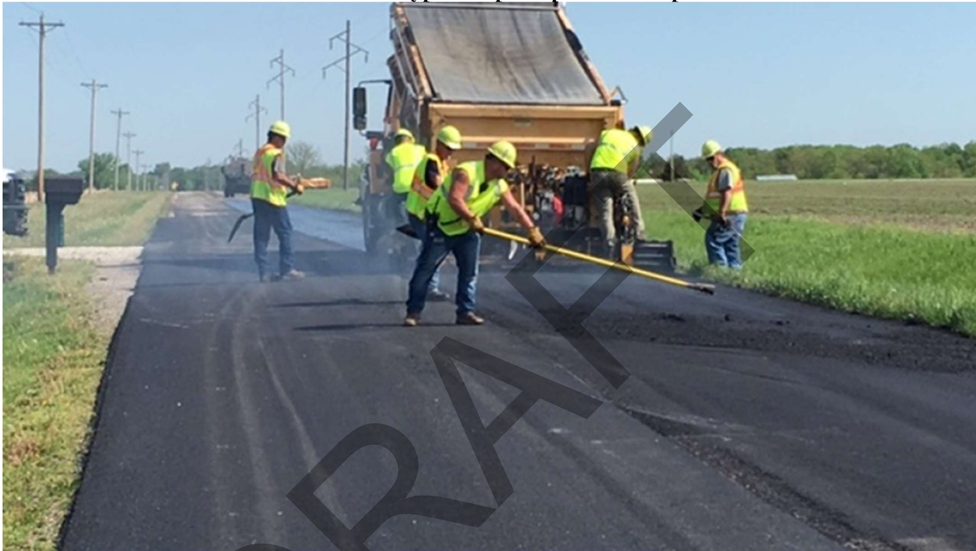
Typical asphalt pavement repair
