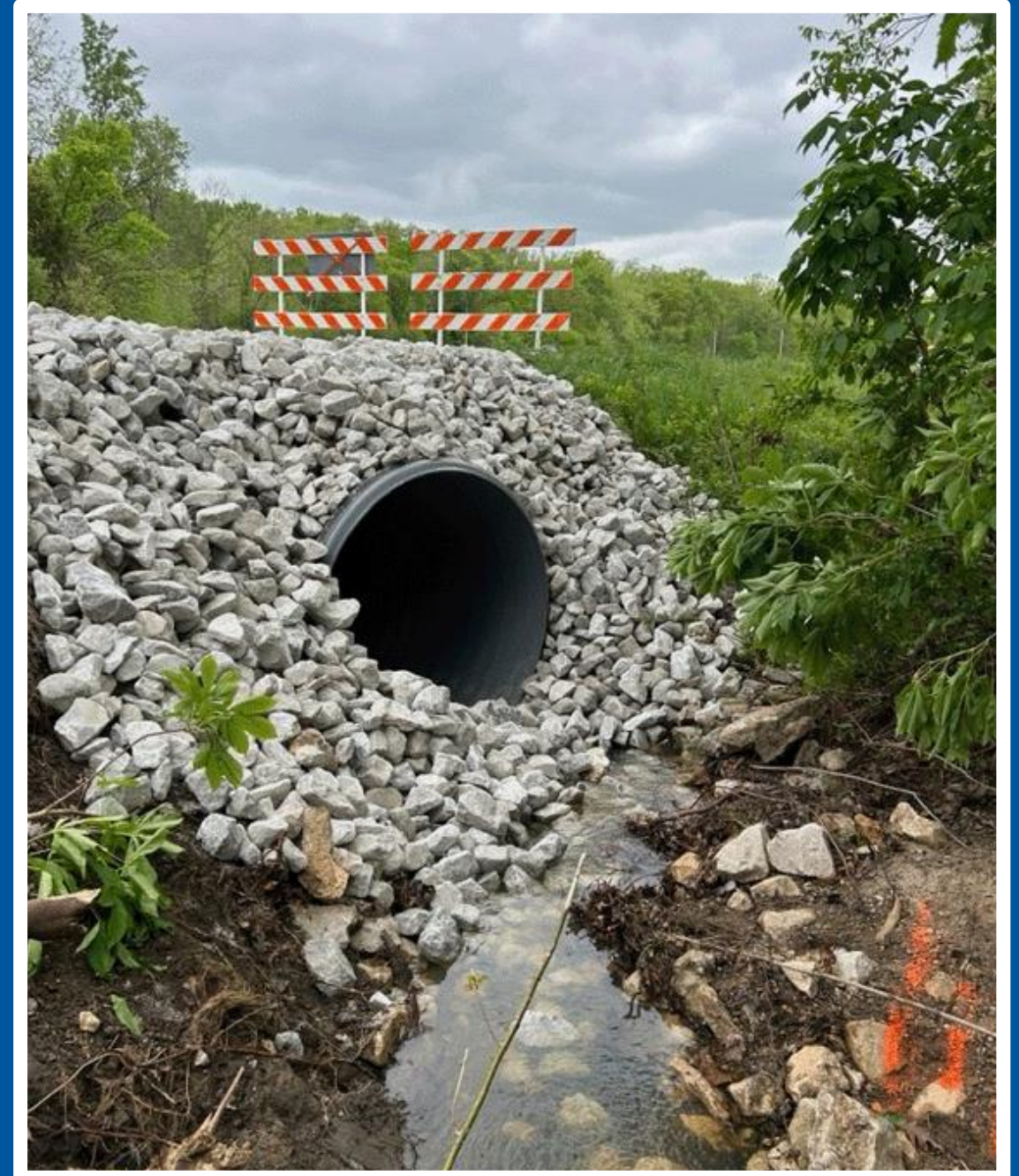
Culvert washout repair on Boone County Route F
