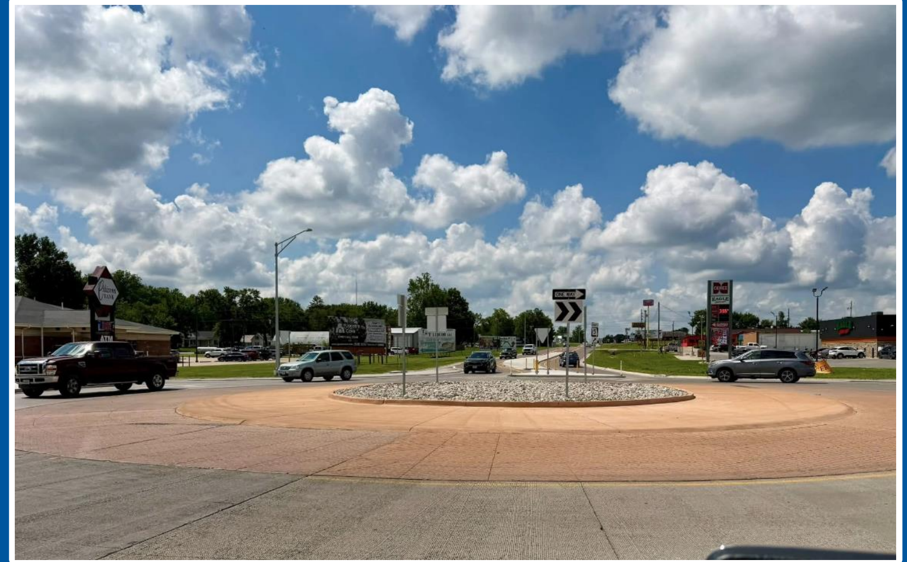
Missouri Routes 5 & 52 Intersection improvements in Versailles
