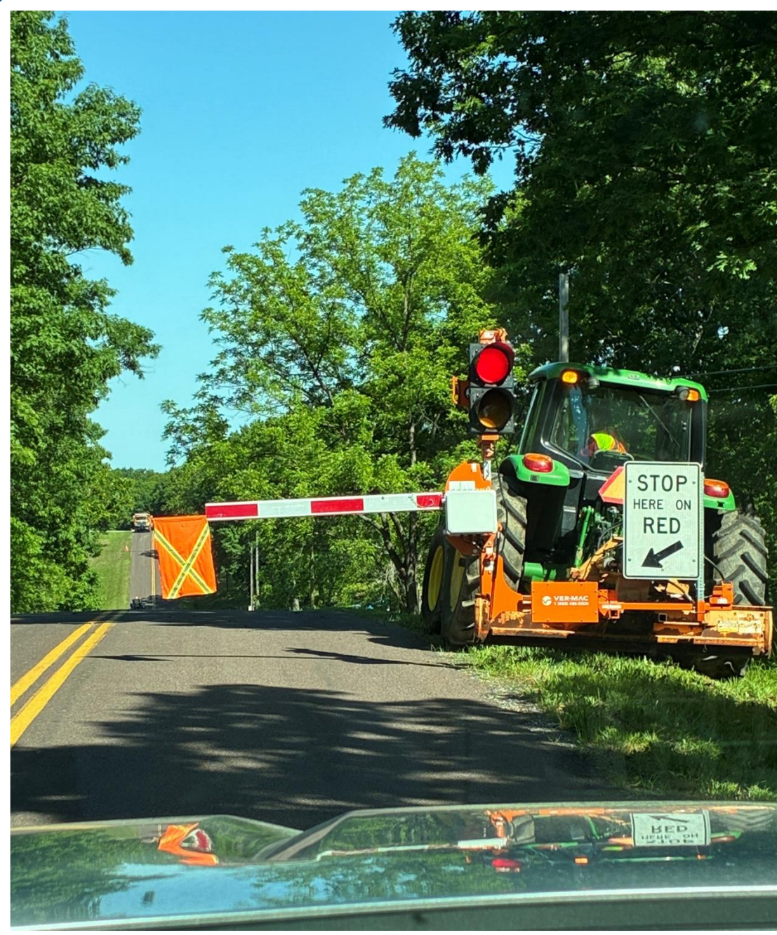
Using a tractor-mounted flagger on Maries County Route M paving operations
