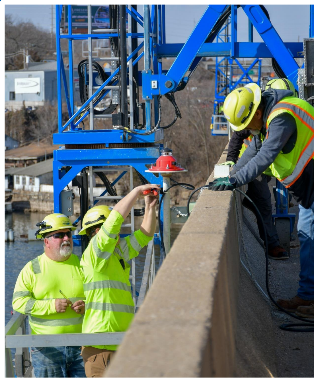
Changing navigation lighting on the Grand Glaize Bridge at Lake of the Ozarks
