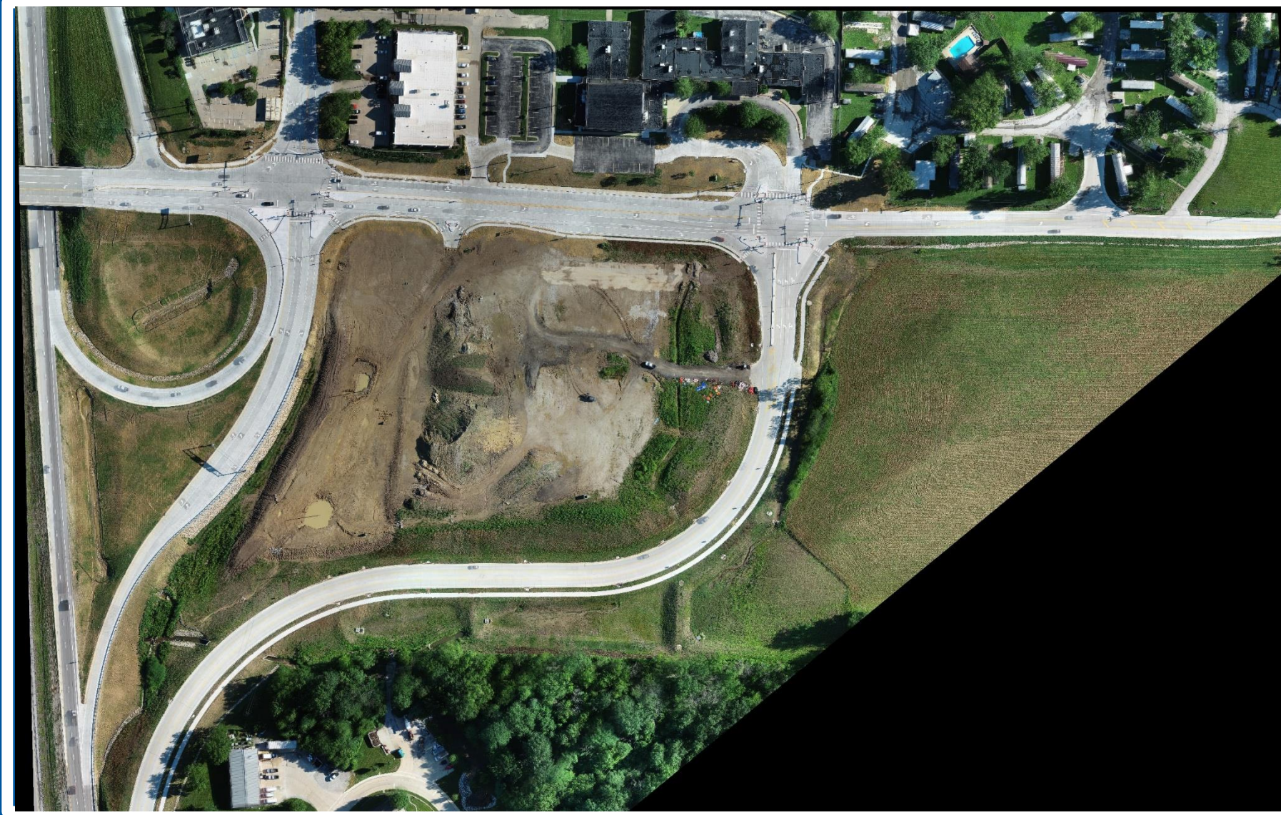
U.S. 63 and Route AC New interchange in Columbia
