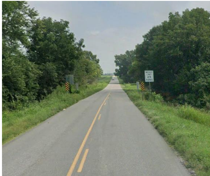
Benton County Route E Culvert Replacement over Barker Creek
