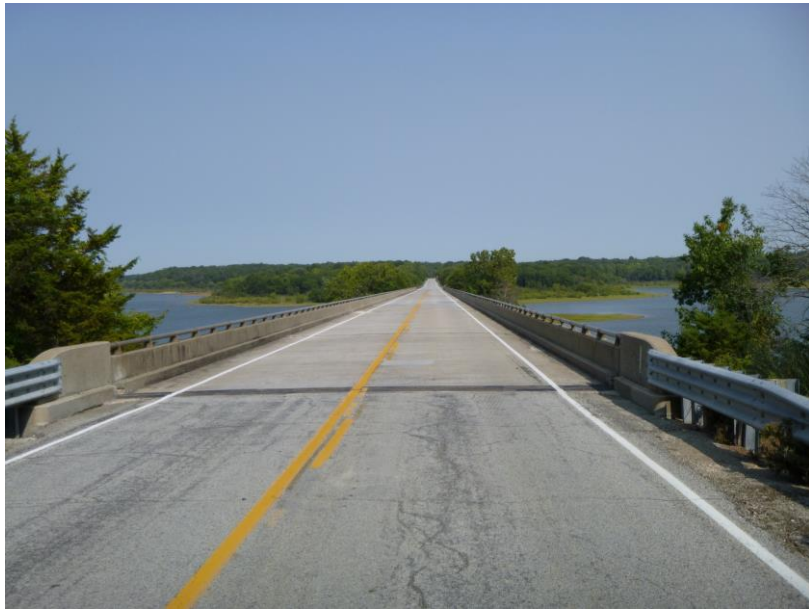
Henry County Route U Bridge Re-Deck over Truman Reservoir
