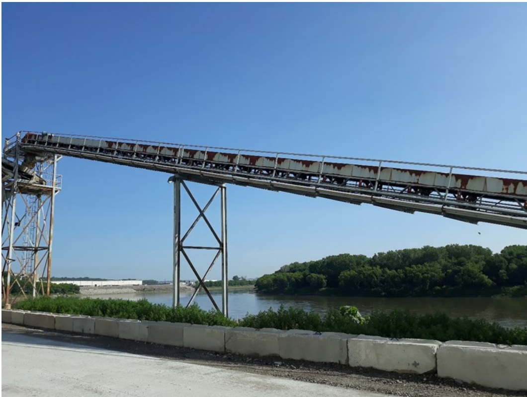
Conveyor Current Condition
