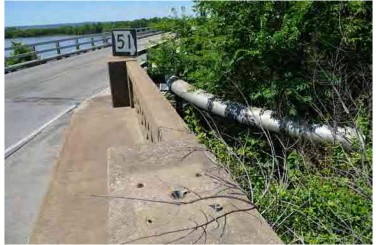
Figure 14 Gas Pipeline on Existing Bridge
