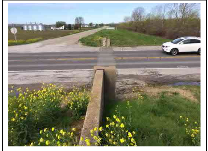
Figure 6 – Gap in Bois Brule levee at Route 51.
