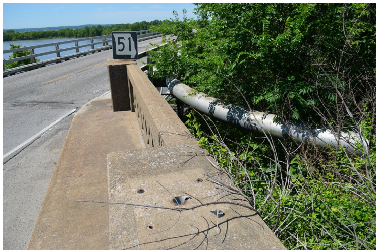
Figure 2-9. Gas Pipeline on Existing Bridge
