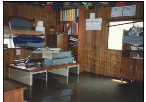
Flooding inside the St. Charles project office.
