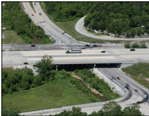
Rehab work on one of 21 bridges on I-55.
