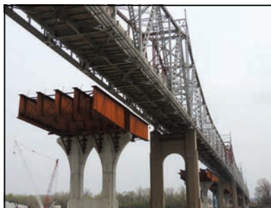
Bridge girders set behind current bridge.
