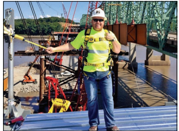
Andy Tuerck during the Boone Bridge construction
